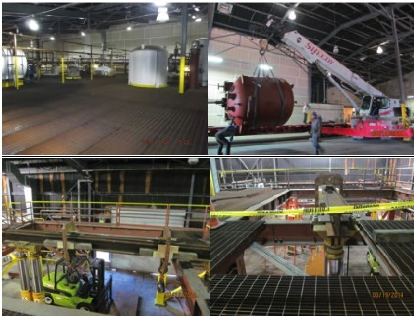
Figure 3: New Reactor Placement and Installation 1
