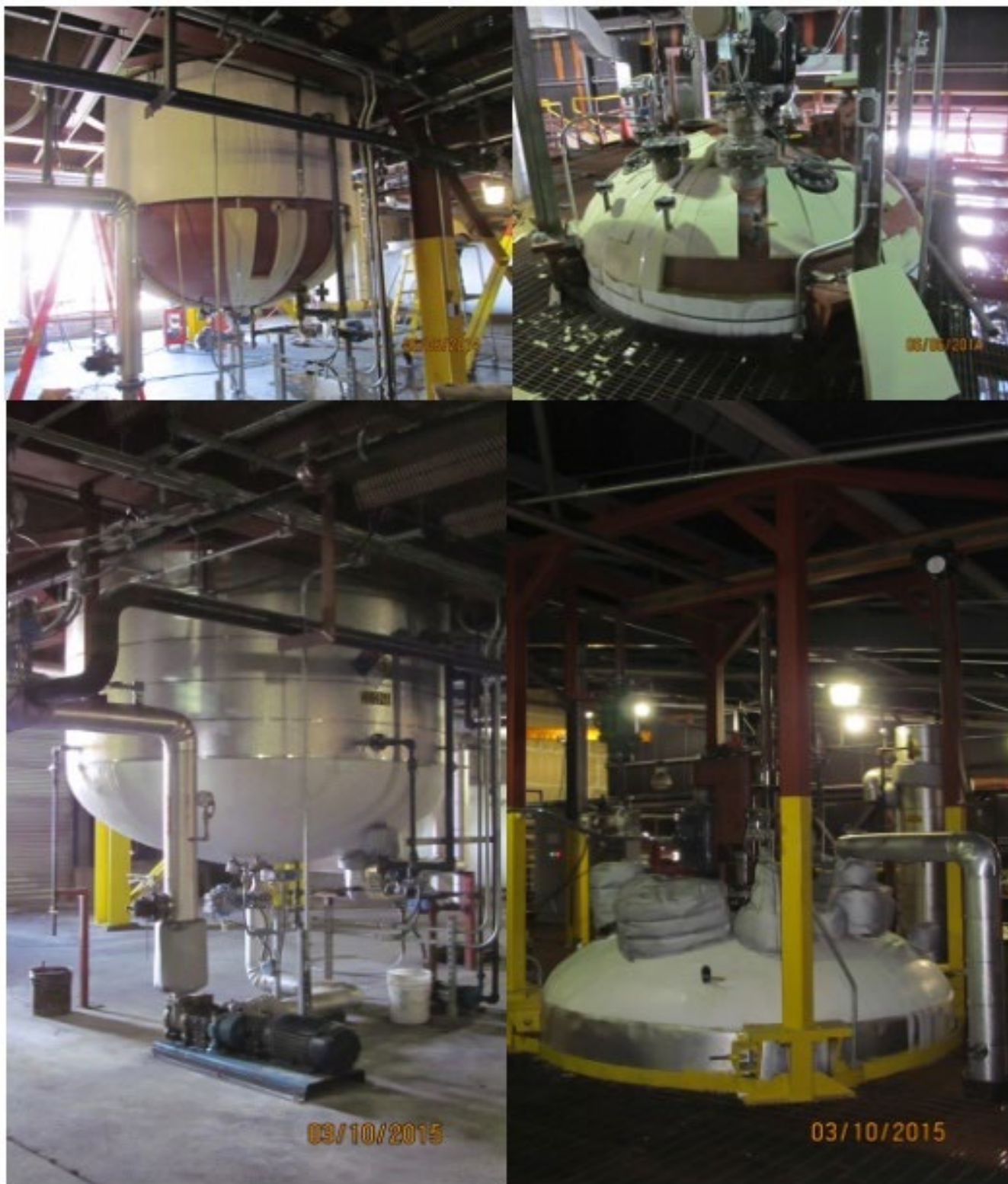
Top Left: Insulation installed on bottom of reactor. Top Right: Insulation installed on top of reactor. Bottom Left: Bottom of reactor fully installed and commissioned. Bottom Right: Top of reactor fully installed and commissioned.
