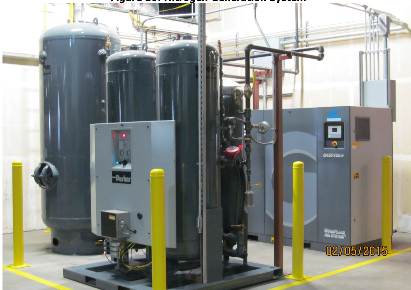
Figure 10: Nitrogen Generation System
