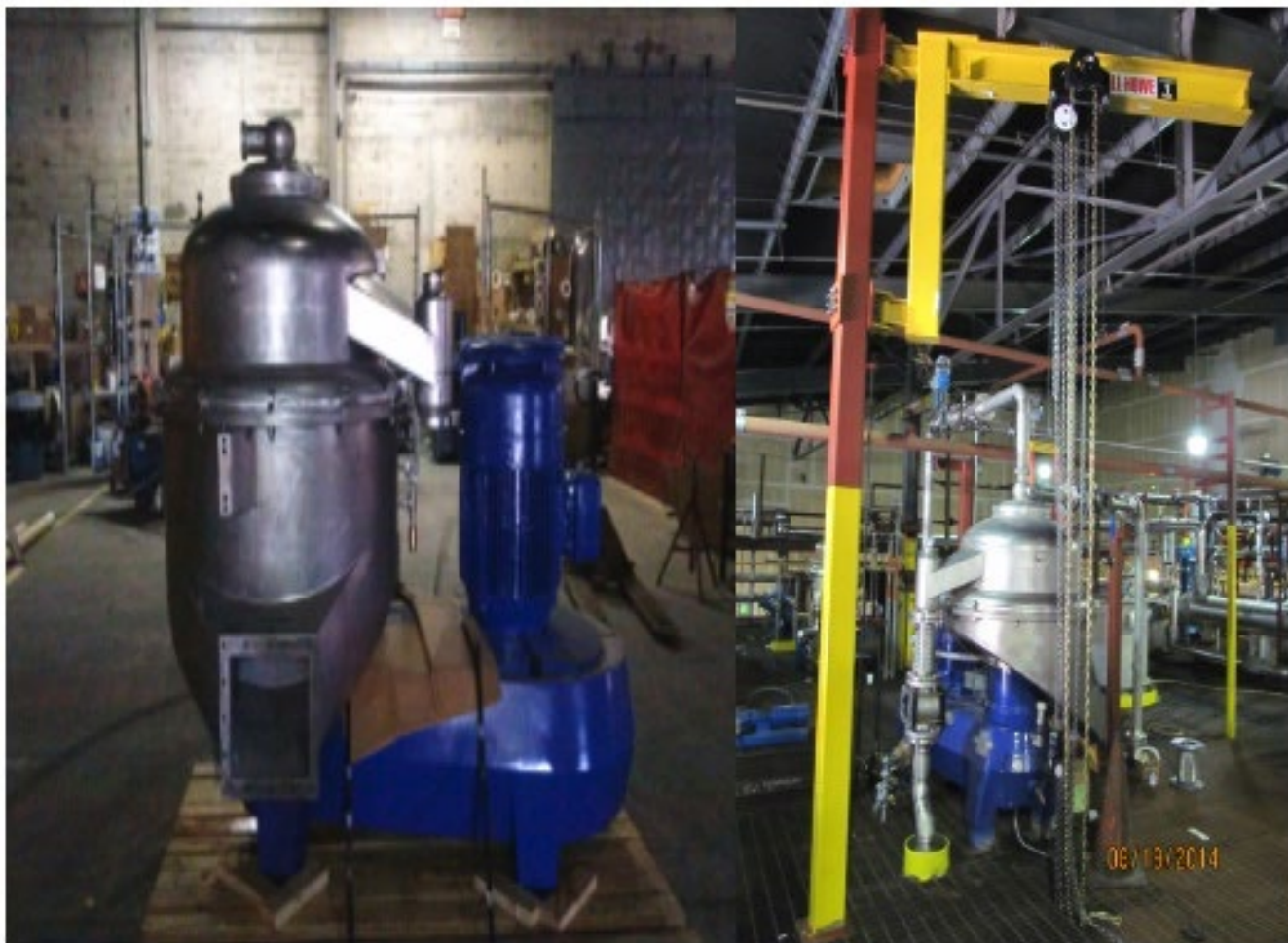
Left: Centrifuge received and prepared for installation. Right: Centrifuge installed in process room and commissioned.
