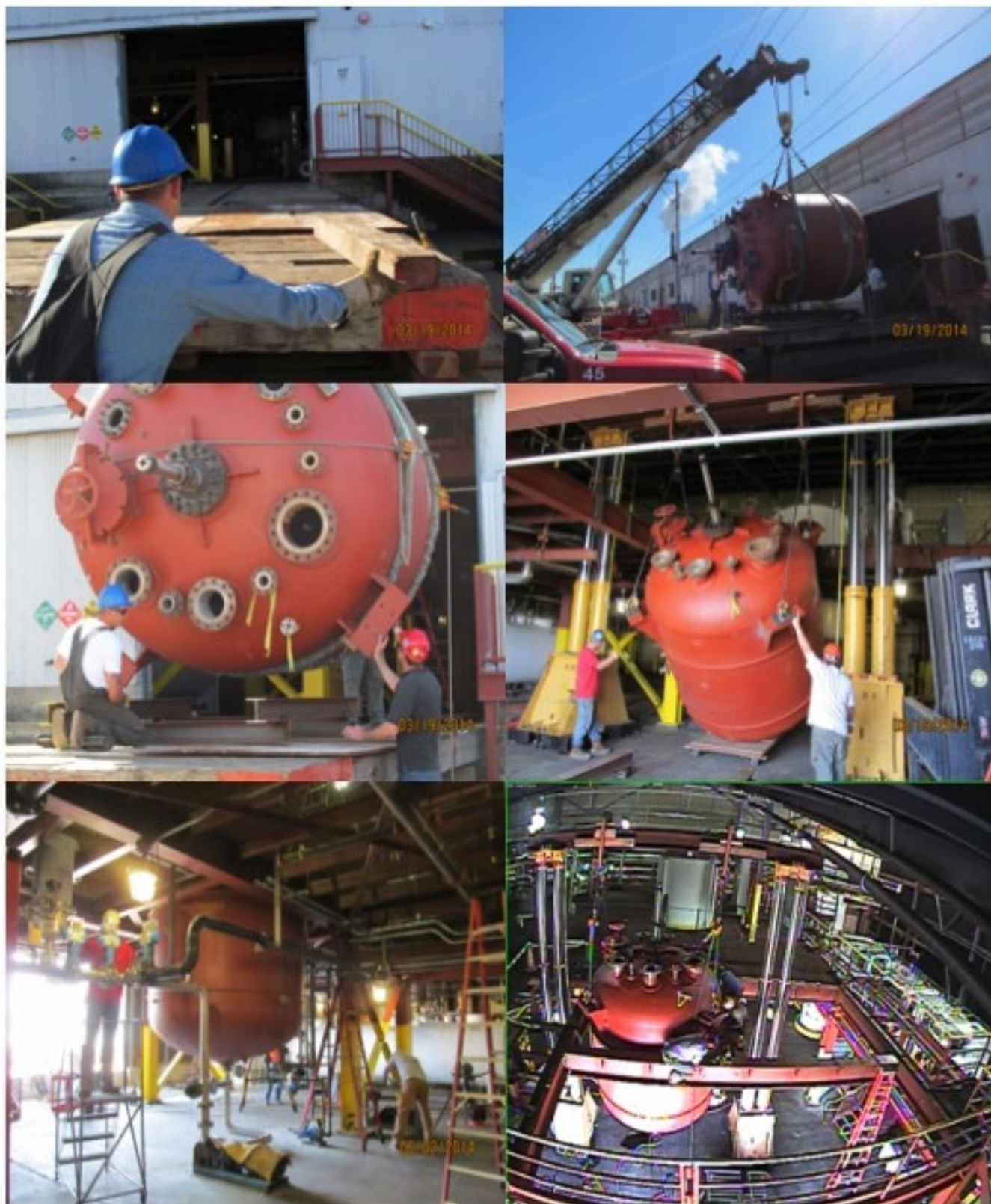
Top Left: Construction of a temporary dock to support reactor transfer. Top Right: Reactor transfer. Middle Left: Placement of reactor on dock. Middle Right: Reactor placement. Bottom Left: Reactor placed, and piping started. Bottom Right: Reactor placed, and piping started.
