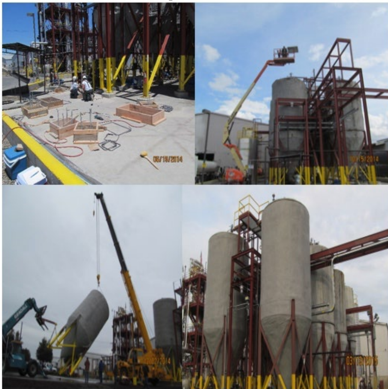
Top Left: Foundations prepared for new tanks. Top Right: Pipe racks and tank supports constructed. Bottom Left: Preparation for tank placement. Bottom Right: Portion of new tanks installed.
