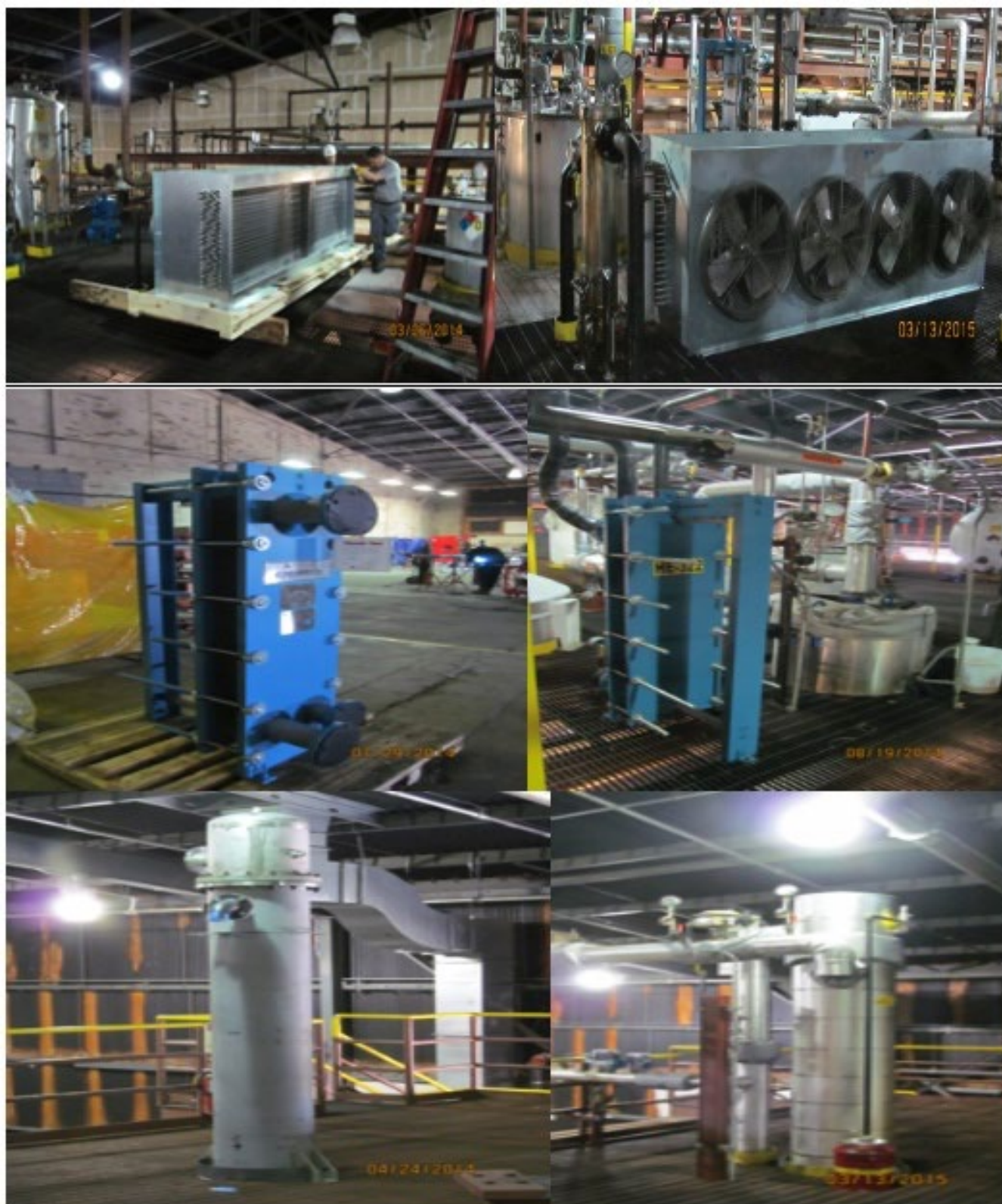
Top Left: Fin fan cooler placed in process room. Top Right: Fin fan cooler fully installed and commissioned. Middle Left: Supercharger received and prepared in warehouse. Middle Right: Supercharger installed in process room and commissioned. Bottom Left: Top of heat exchanger prior to piping, insulation and ancillary equipment. Bottom Right: Top of heat exchanger installed and commissioned.
