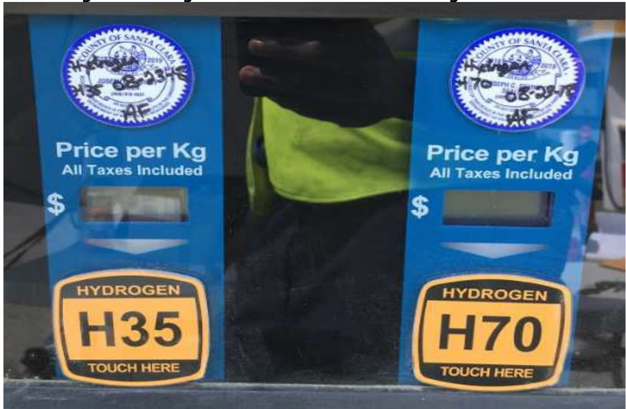
Figure 15: Weights and Measures Labels Showing Certification
