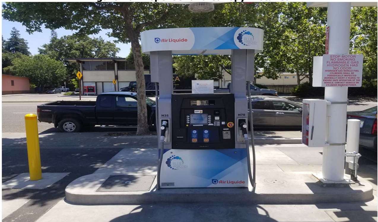
Figure 16: Dispenser and Canopy Installed
