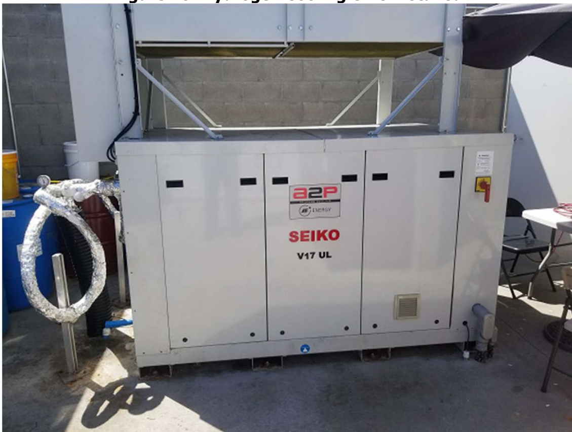
Figure 10: Hydrogen Cooling Unit Installed
