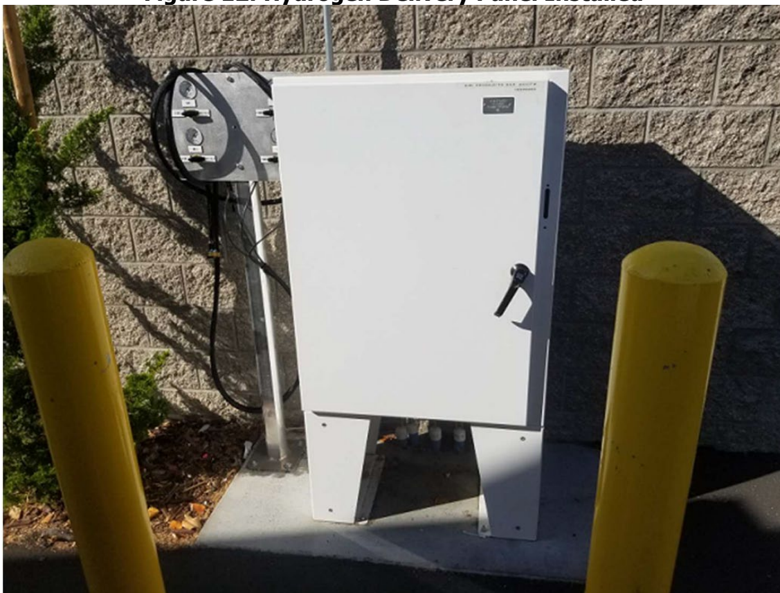
Figure 12: Hydrogen Delivery Panel Installed
