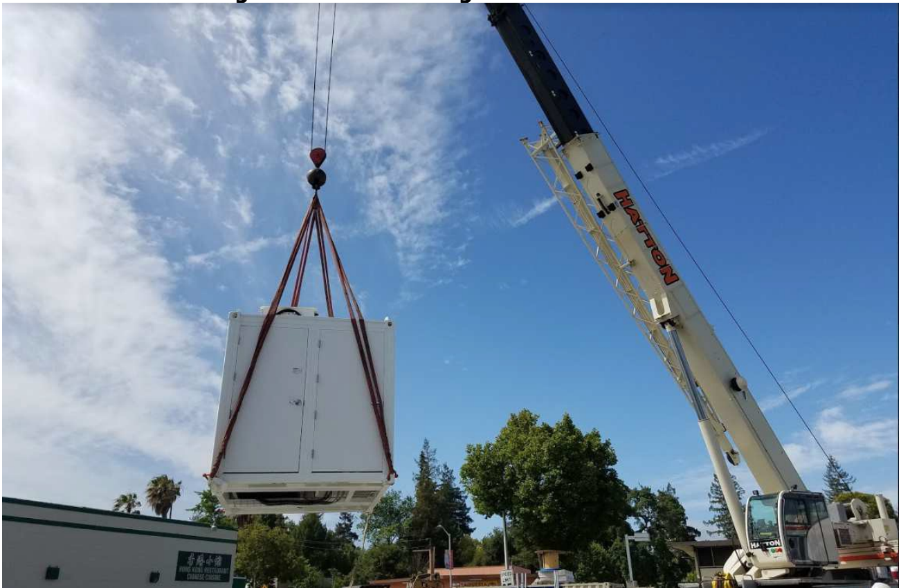
Figure 5: Crane Setting Skids into Position
