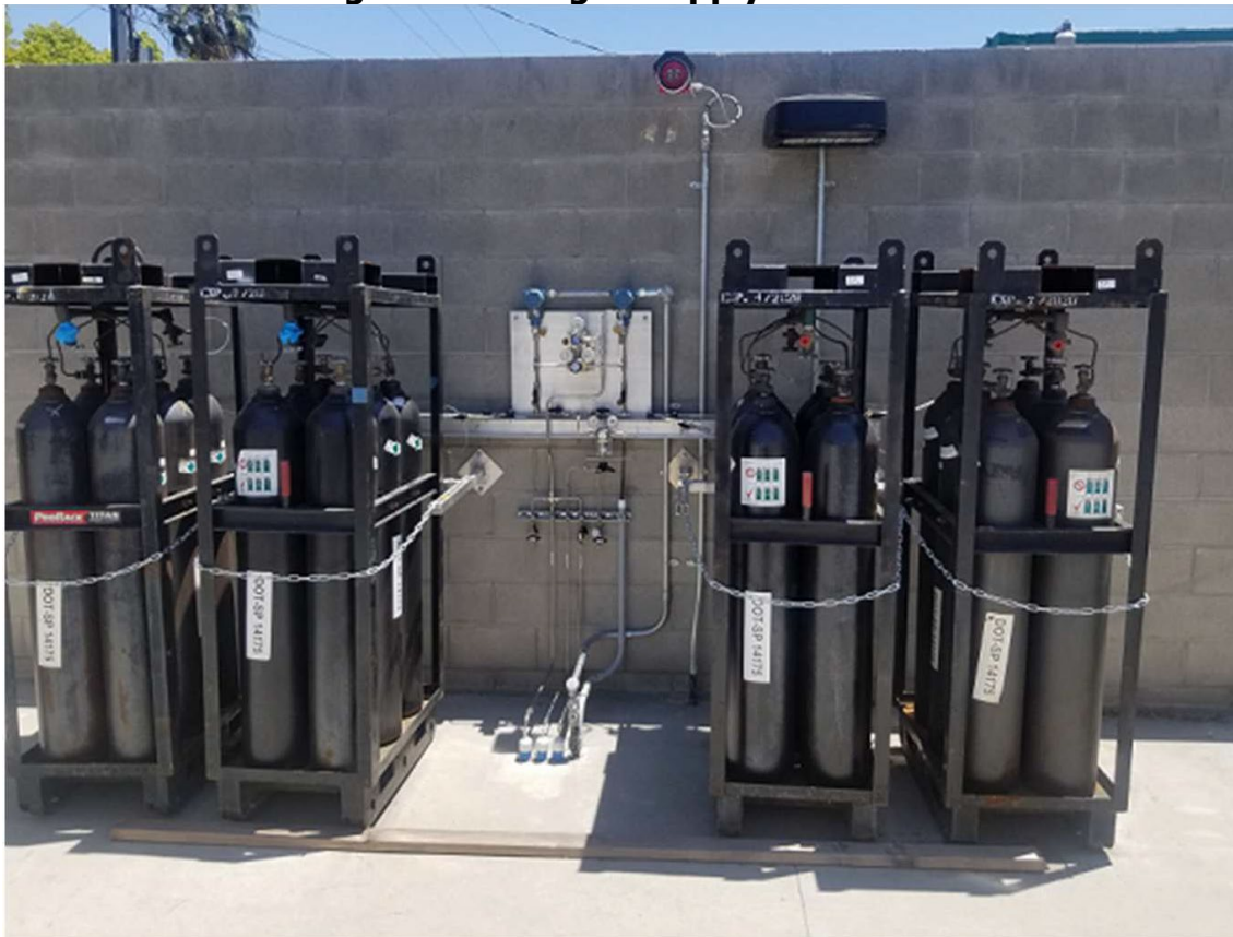
Figure 9: Nitrogen Supply Installed
