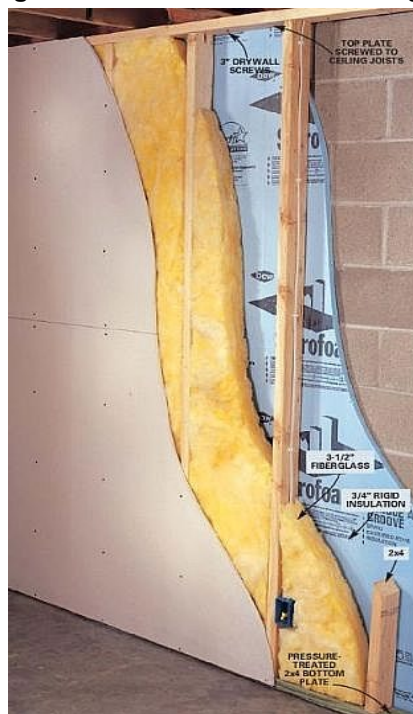
Figure 3-4: Brick Wall with Furring Details
