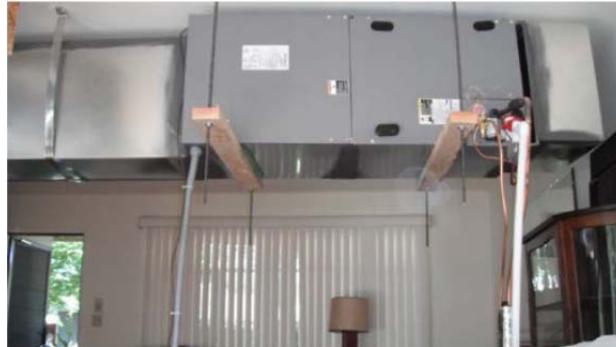
Figure 5: Reference Cooling System Installed in the Research Home
