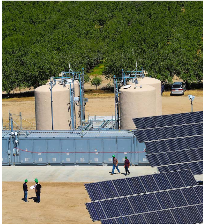
Figure 24: EnerVault Flow Battery Integrated with Photovoltaic System in Turlock
