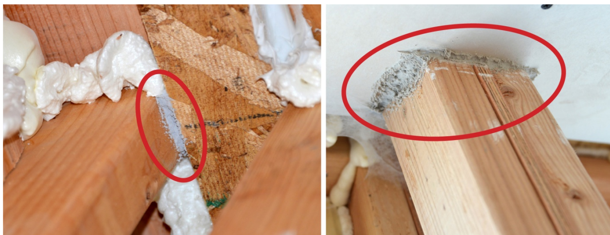
Sealed leak in between manual caulk application at the Honda Smart Home
