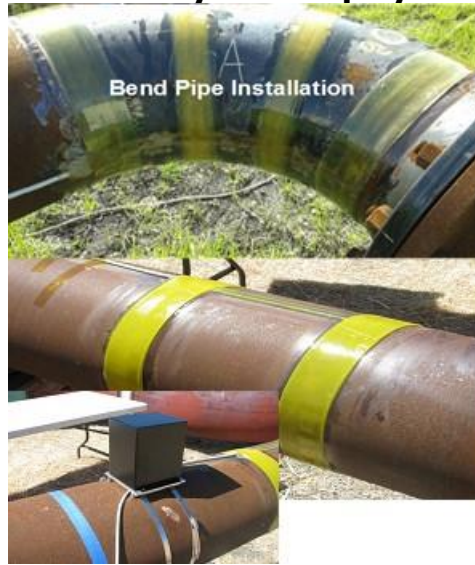
Top: bend pipe installation, bottom: straight pipe installation
