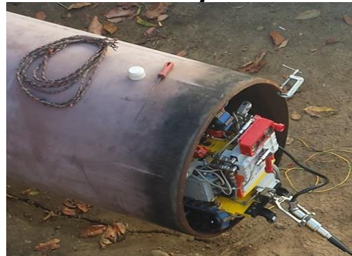
Figure 10: Diakont's Robotic Operational Defect Inspection System (RODIS) at Pipeline Entry
