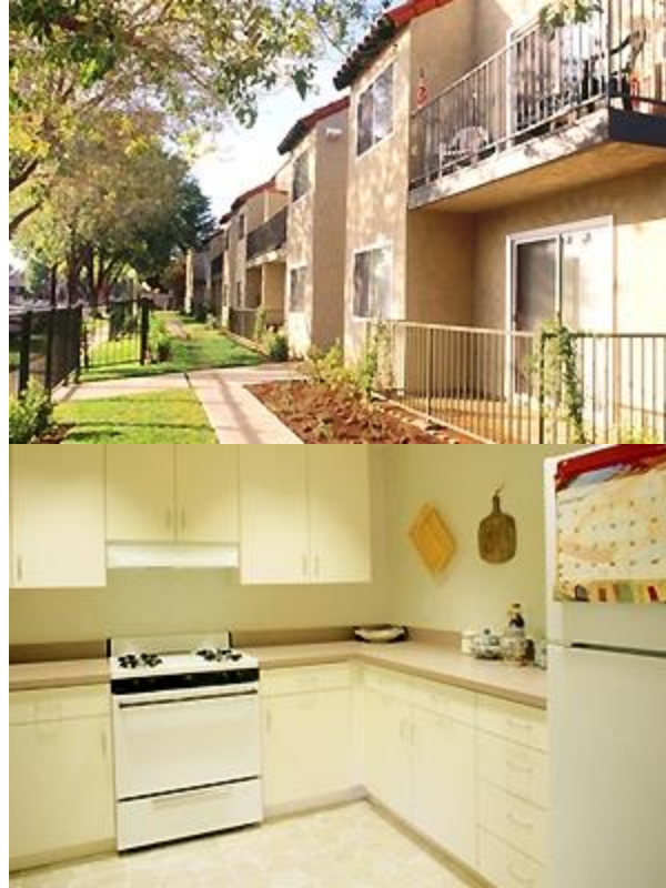
Figure 18: The Village at Beechwood Low-Income Housing Demonstration Site in Lancaster, California
