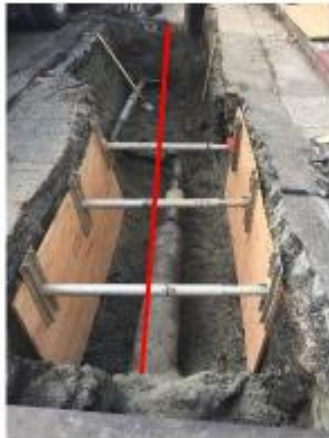
Picture of trench with shoring more main uncovered
