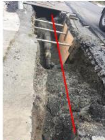
Picture of trench with shoring
