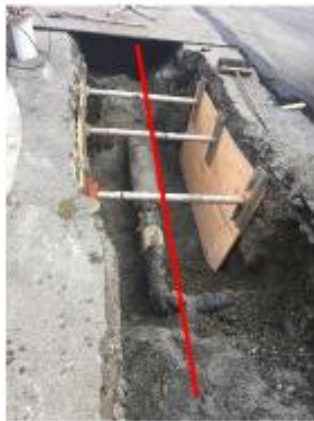
Picture of trench with shoring
