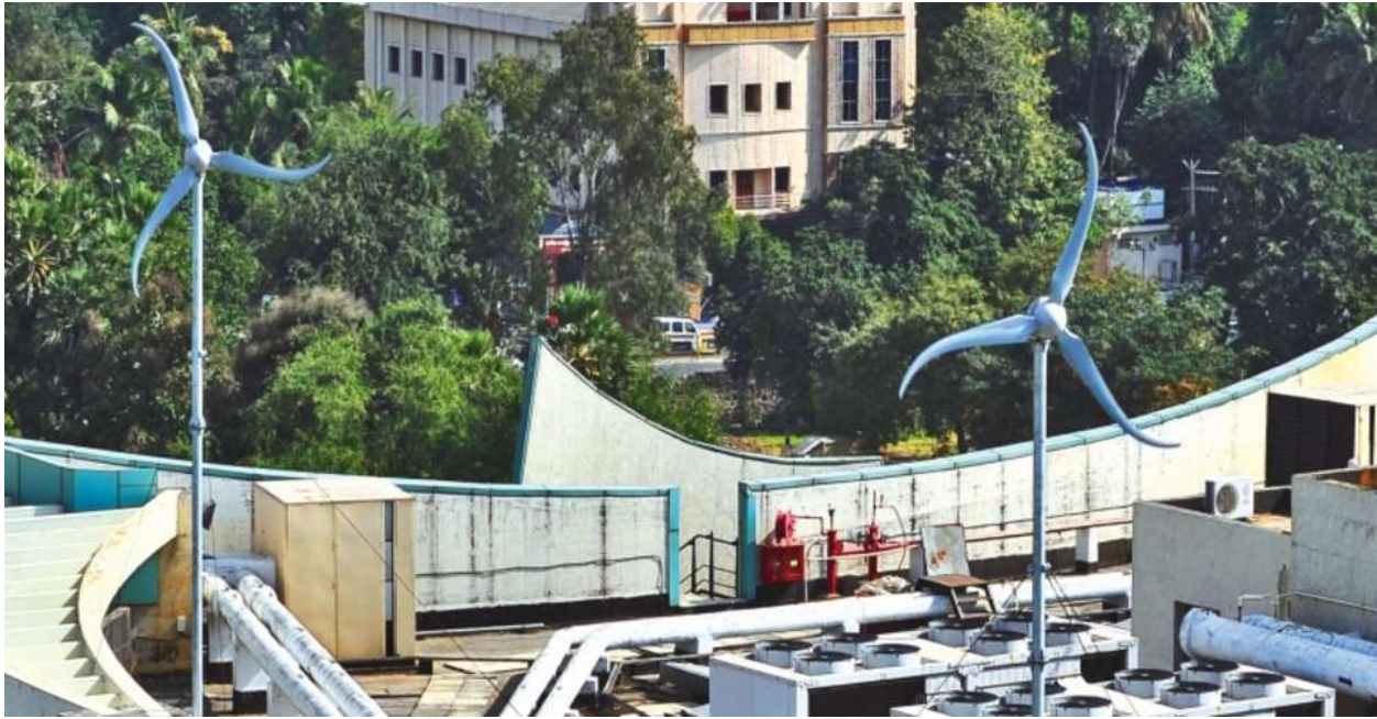
Figure 22: L&T Chennai Campus Micro-Wind Turbines
