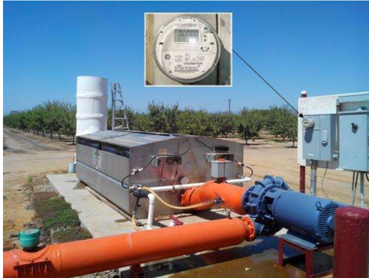
Figure 10: Example of Smart Meter at a Pumping Station for Irrigation at an Almond Orchard
