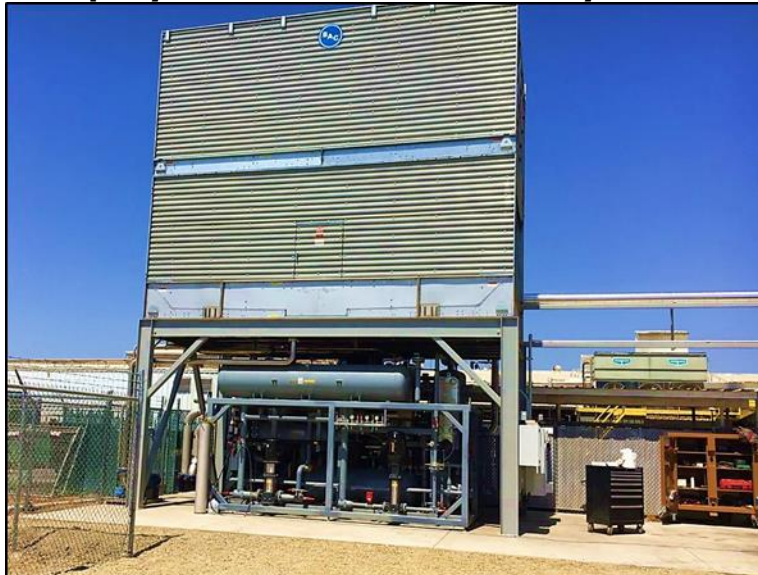
Figure 7: Cooling Towers Above the Absorption Chiller at the Gallo Cattle Company Cheese Production Facility in Atwater, California
