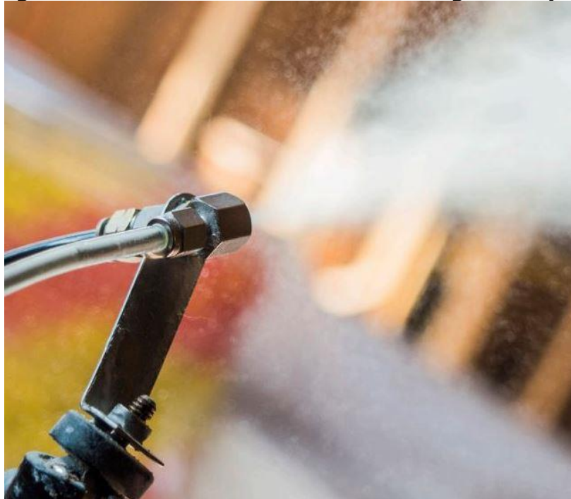
Figure 4: AeroBarrier Sealant for Building Envelopes
