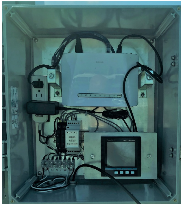
Figure B-7: Transformer Management System Internal Components
