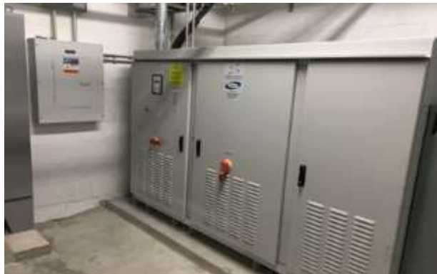
Figure 10: Interior of Inverter Room Showing BIGI250™ and Electrical Systems
