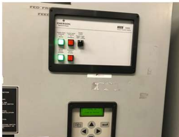
Figure 30: Automatic Transfer Switch-1 Life Safety Returned to Normal Operation
