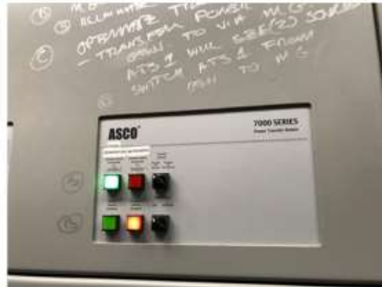
Figure 29: Manual Transfer Switch Status Prior to Transfer of Power Back to Grid-tied
