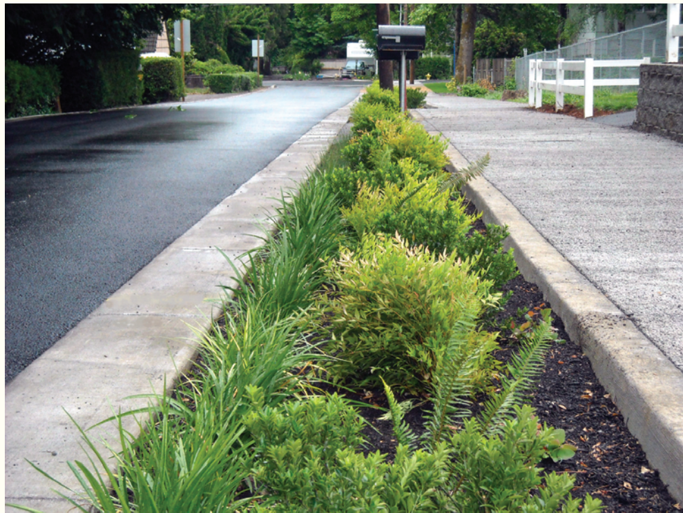
This residential street in Milwaukie, Oregon has no curbs, just a concrete border. Polluted runoff sheets off the road into the planter where it is filtered. Photo courtesy of Kevin Robert Perry.
