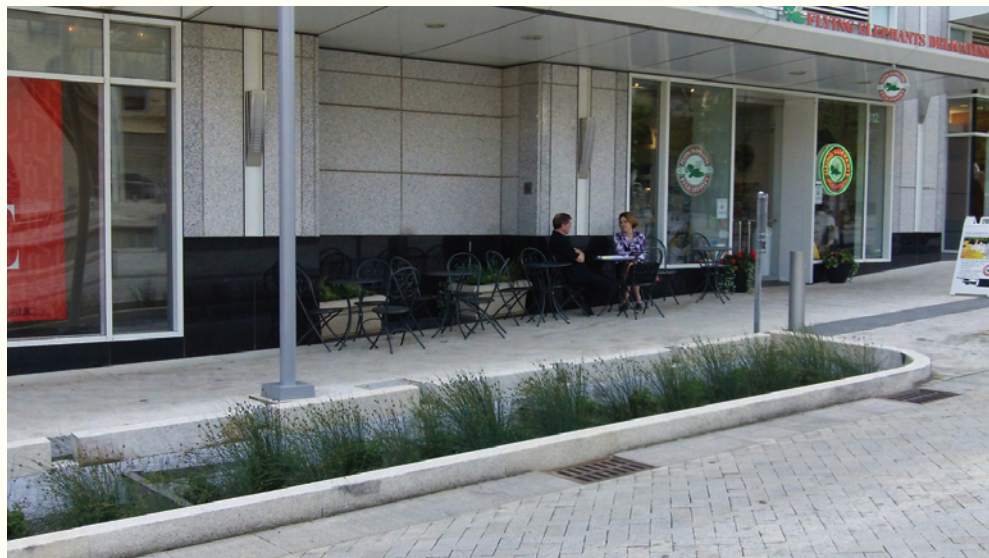
In downtown Portland, a planter adds greenery to the streetscape while treating stormwater. Photo by Lisa Owens Viani.
