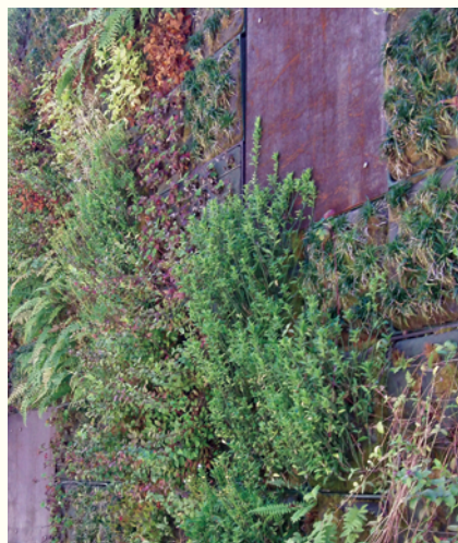
Green walls like this one at a motel in Portland, Oregon can slow and filter runoff from roofs. Photo by Lisa Owens Viani.
