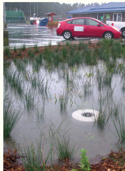
This rain garden in Daly City treats polluted water from an adjacent parking lot. Photo above and below by SFEI.
