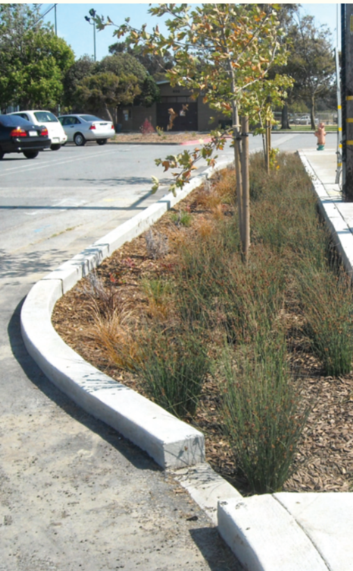
Stormwater from the street flows into this curb extension in San Bruno.
