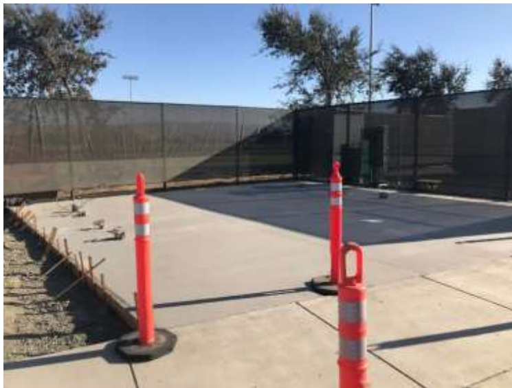
Figure 26: Battery Energy Storage System Equipment Pad
