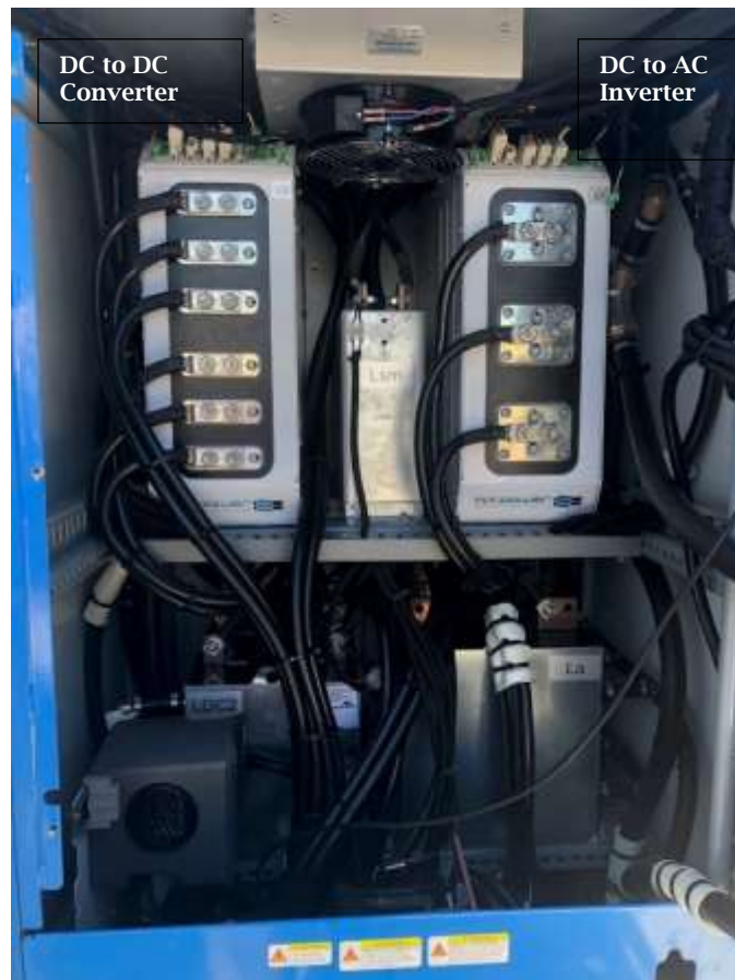
Figure 15: Photo of Internal EPC Power Corporation Inverter Cabinet
