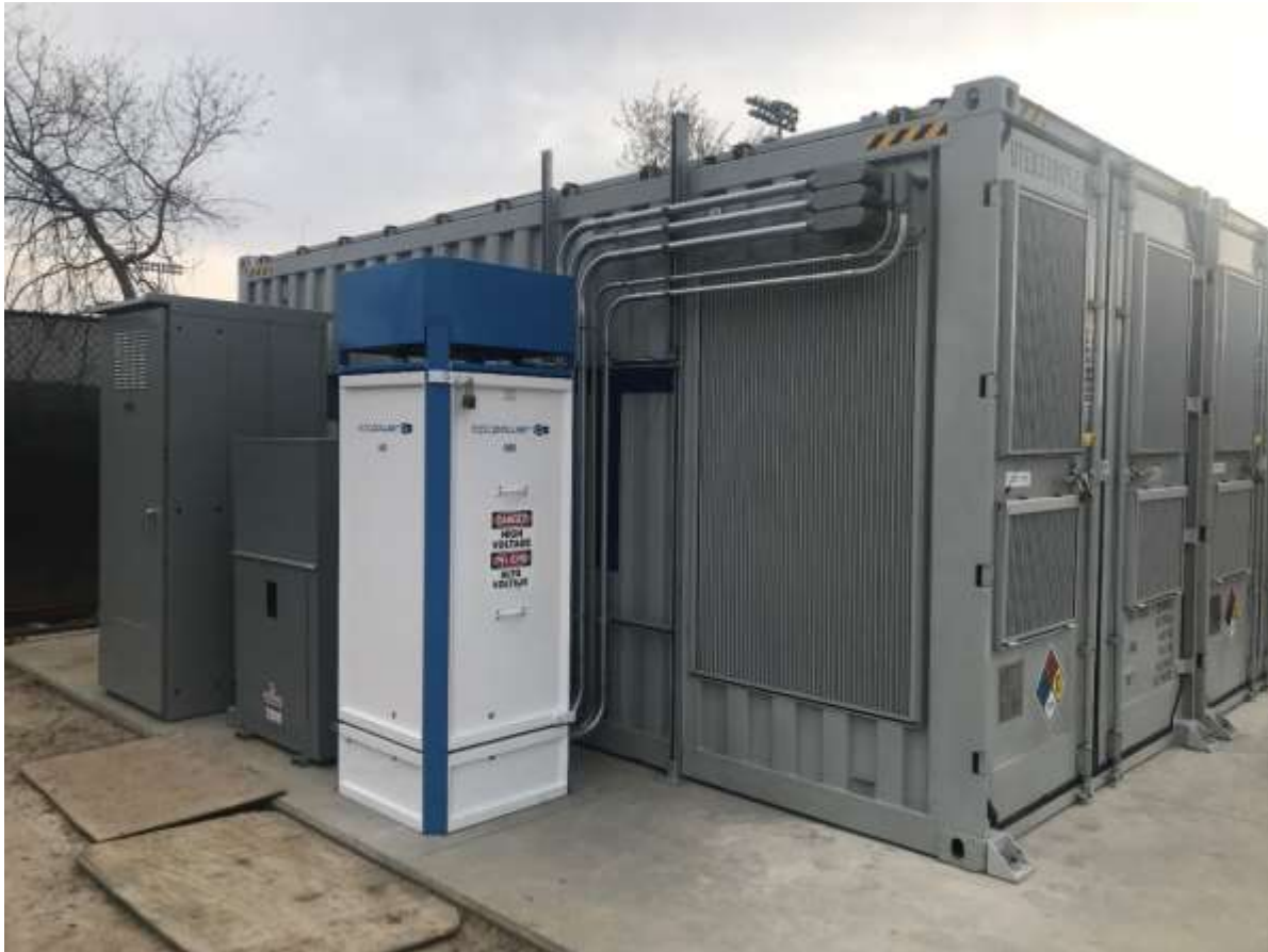
Figure 24: Electrical Systems Installation
