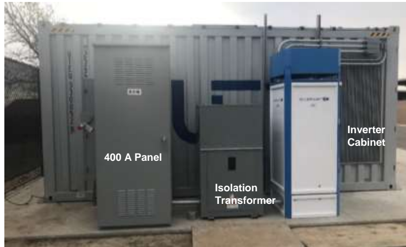
Figure 27: Completed Equipment Installation
