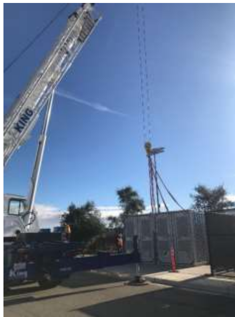
Figure 19: Setting UniEnergy Technologies Battery Units
