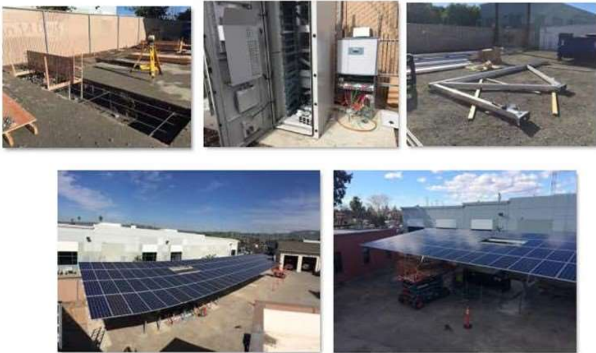
Figure 24: Fire Station 7 Construction Progress and Final Deployment
