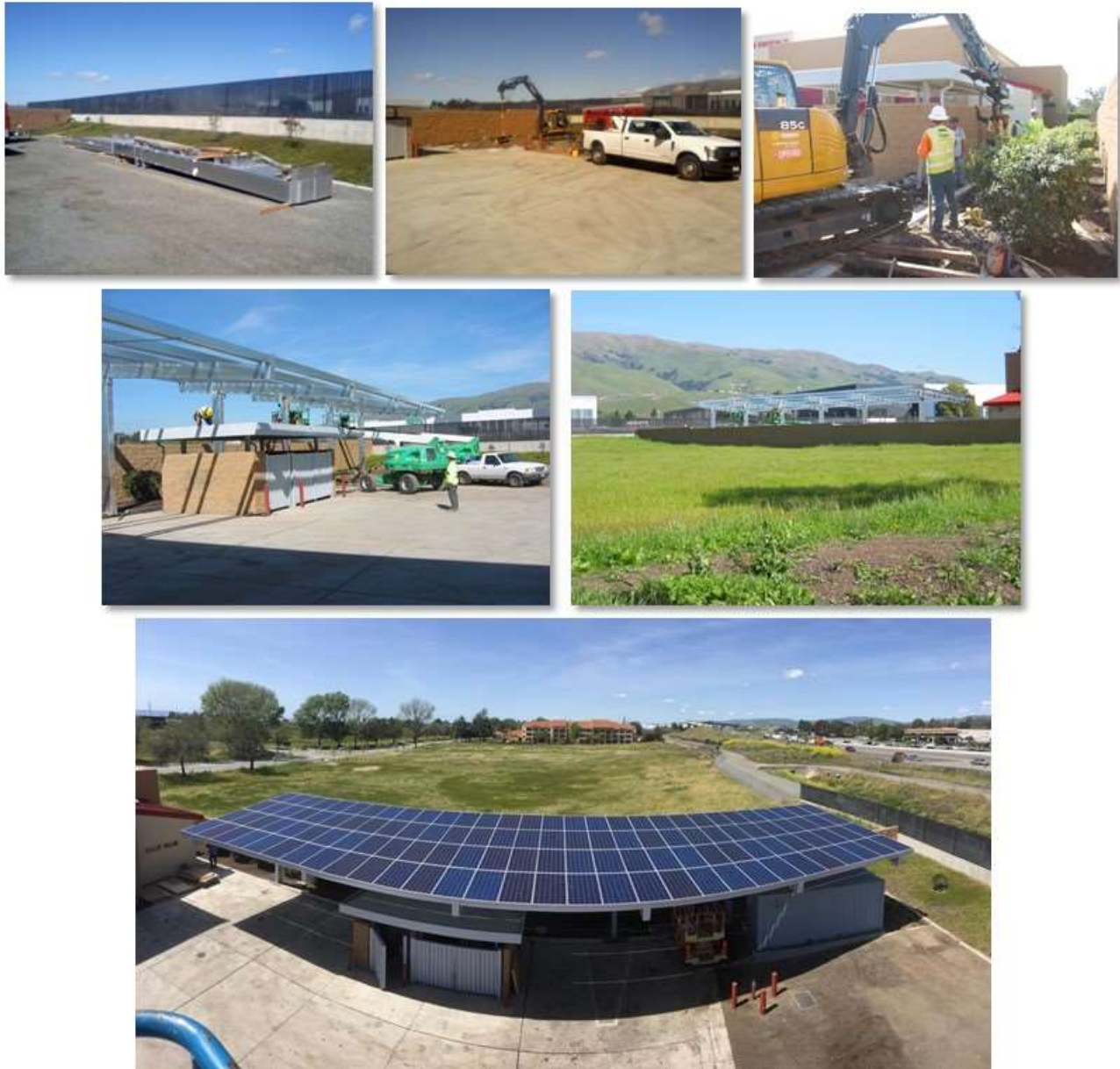
Figure 22: Fire Station 11 Microgrid Construction and Final Deployment
