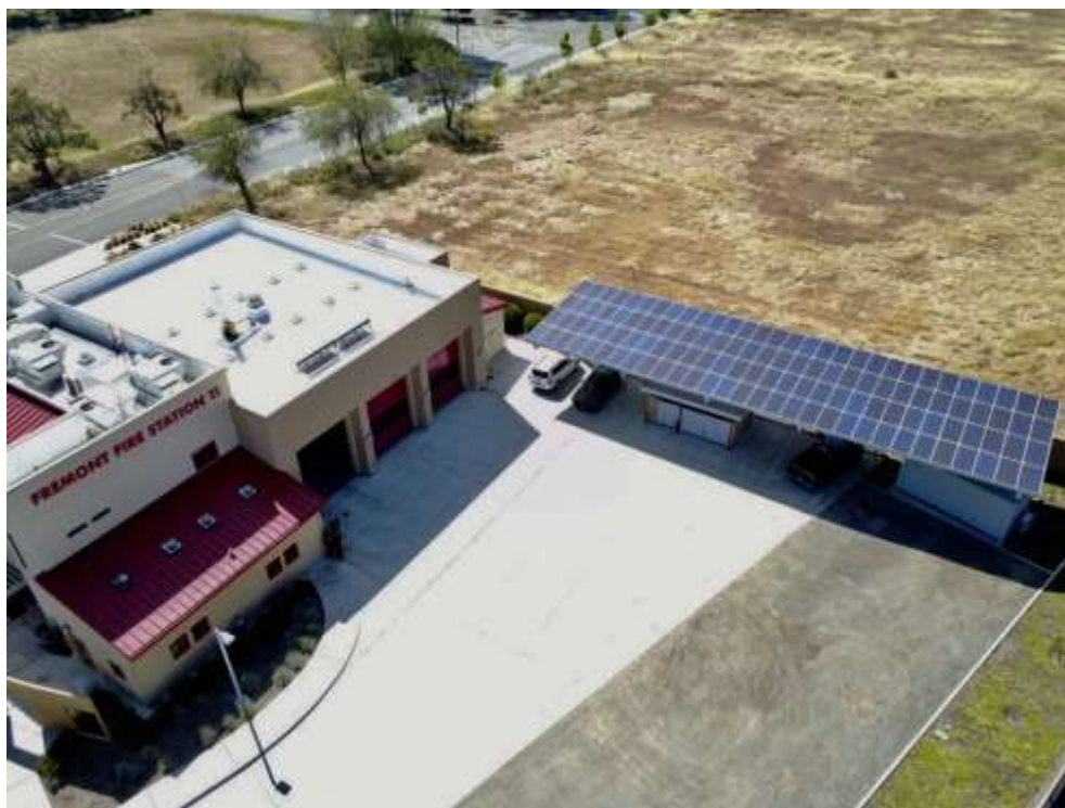
Figure 10: Aerial View of Fire Station 11 Microgrid
