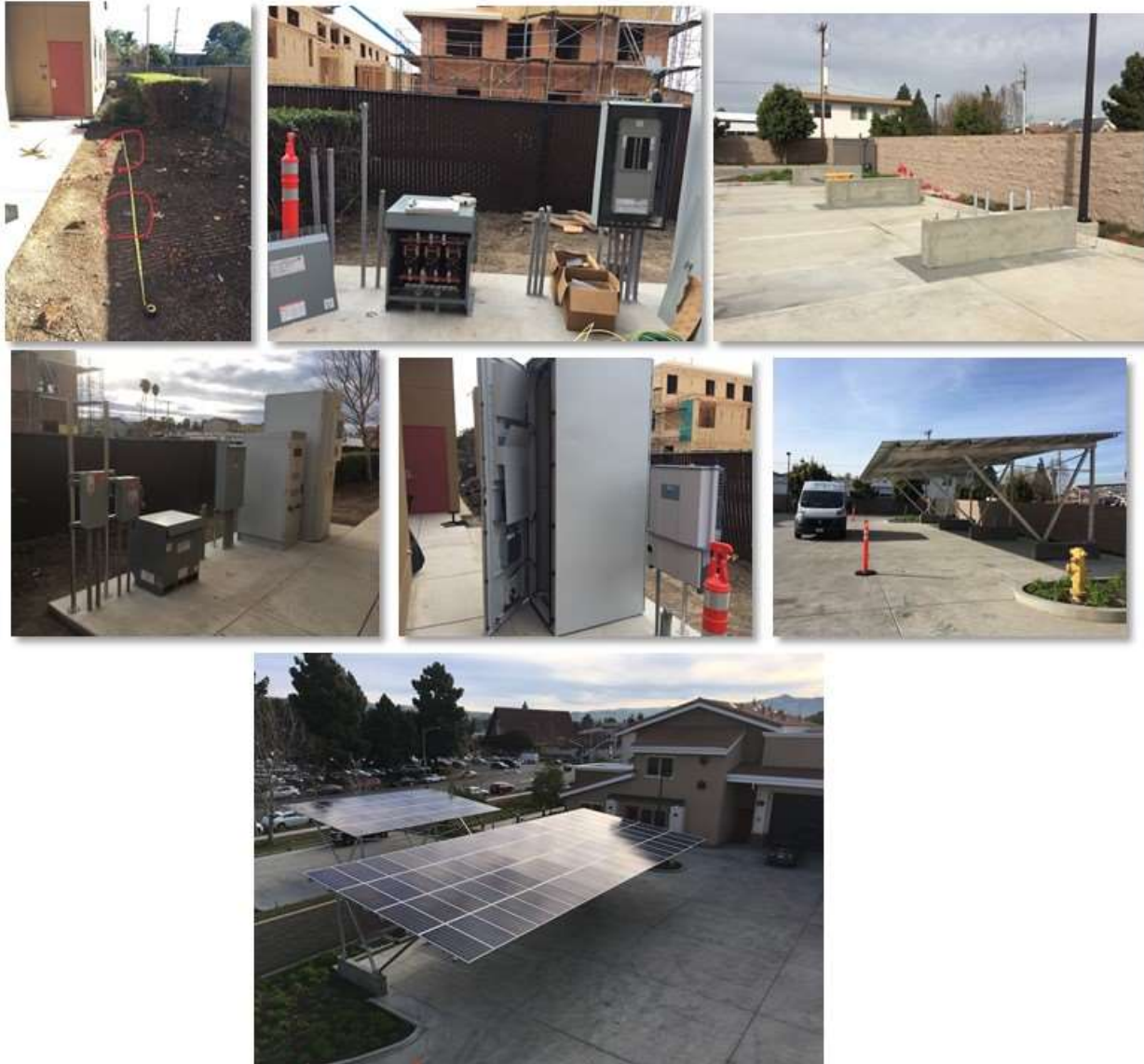
Figure 23: Fire Station 6 Construction Progress and Final Deployment
