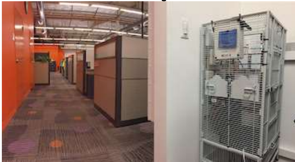
Figure 21: Carbon Dioxide Sensor Package Tested in a General Office Space
