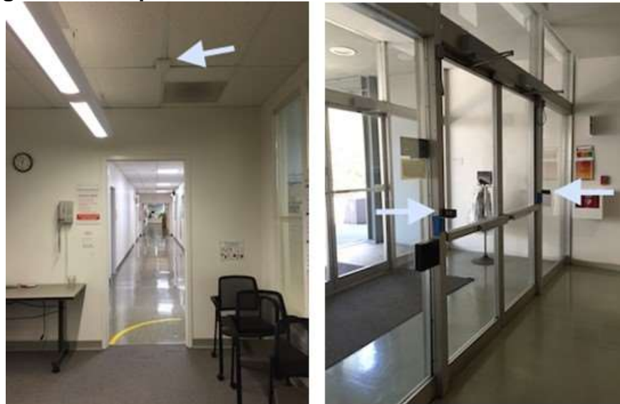
Figure 29: People Counters Tested at Two Different Doorways
