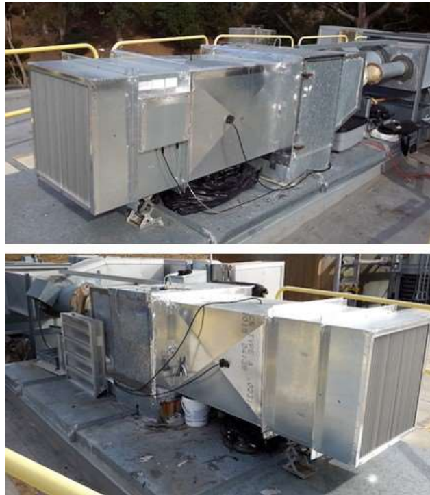
(Top) EAMS installed with a vertical-blade louver. (Bottom) The horizontal-blade louver is shown on the side of the system being tested.
