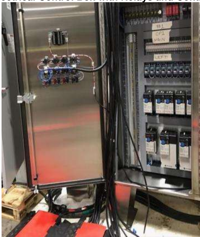
Figure 20: Main Electrical Control Box with Relays and Control Units of System
