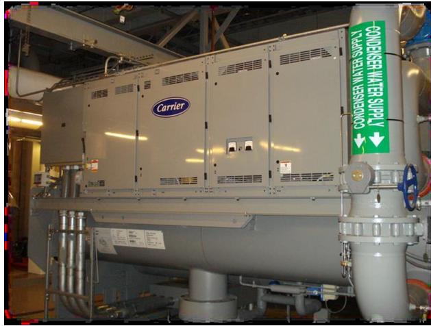
Figure 12: Chiller at Pharmaceutical Host Site
