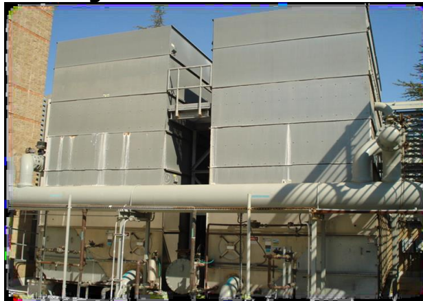
Figure 11: Cooling Towers at Pharmaceutical Host Site
