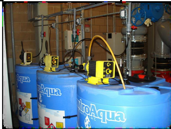
Figure 21: Cooling Tower Chemical Feed System at Pharmaceutical Site
