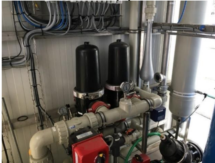
Figure 15: Installed IVG-CT Equipment at Hotel Host Site
