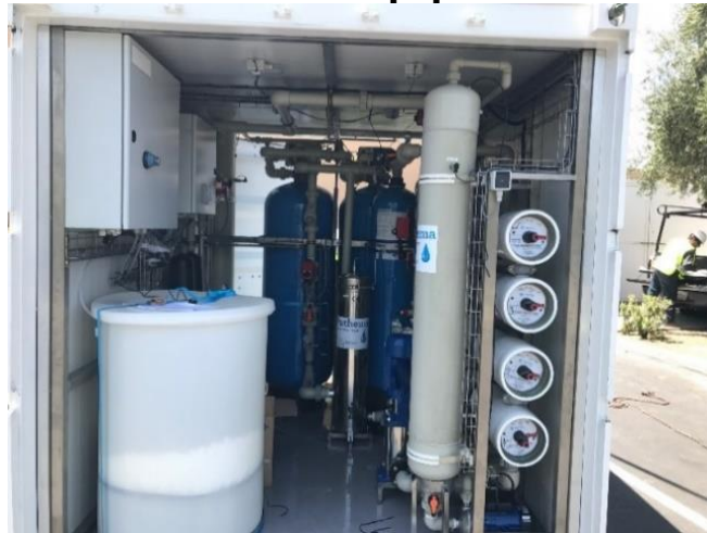
Figure 14: Installed IVG-CT Equipment at Hotel Host Site
