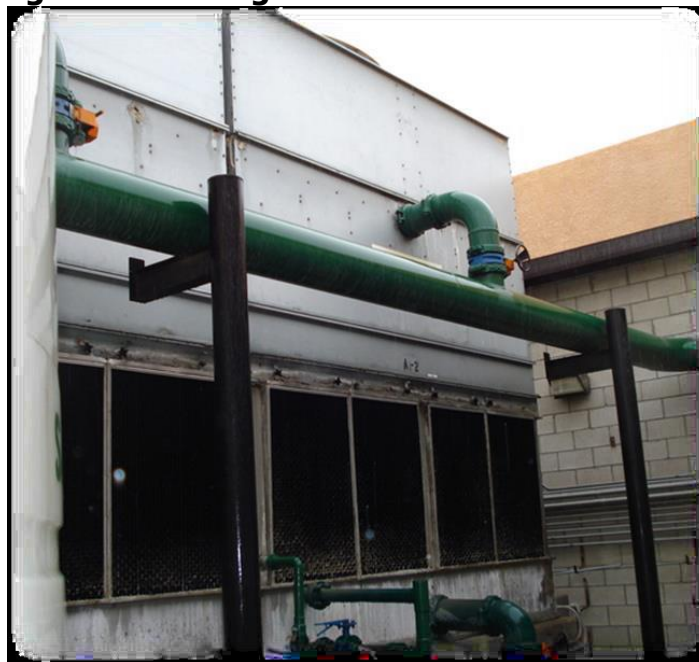
Figure 9: Cooling Tower in Hotel Host Site
