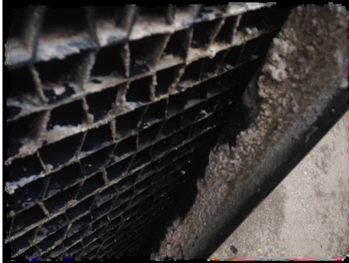
Figure 10: Close-Up of Cooling Tower at Hotel Host Site
