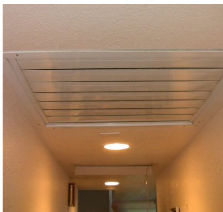
Figure 4-38: Whole-House Fan With Barometric Damper
