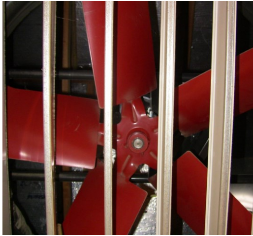
Figure 4-39: Open Barometric Damper With Fan Above
