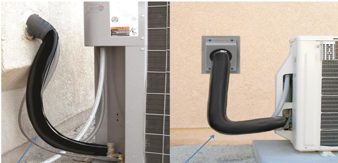
Figure 4-1: Refrigerant Line Insulation
