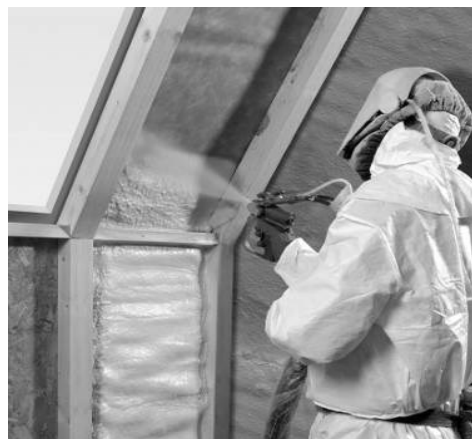
Figure 3-18: Closed-Cell SPF Installation in a Wall Cavity
