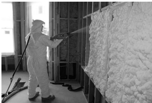
Figure 3-17: Open-Cell SPF Installed in Wall Cavity
