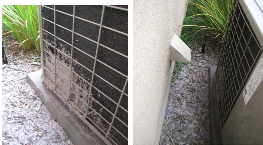
Figure 4-2: Noncompliant Condensing Unit Clearance From Dryer Vents
