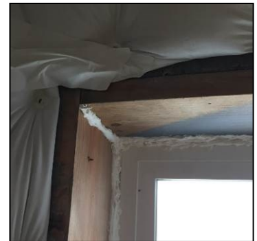
Figure 3-10: Air Sealing
