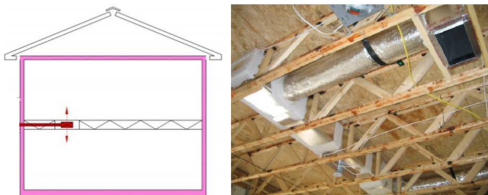
Figure 4-13: Open Web Floor Truss Example
