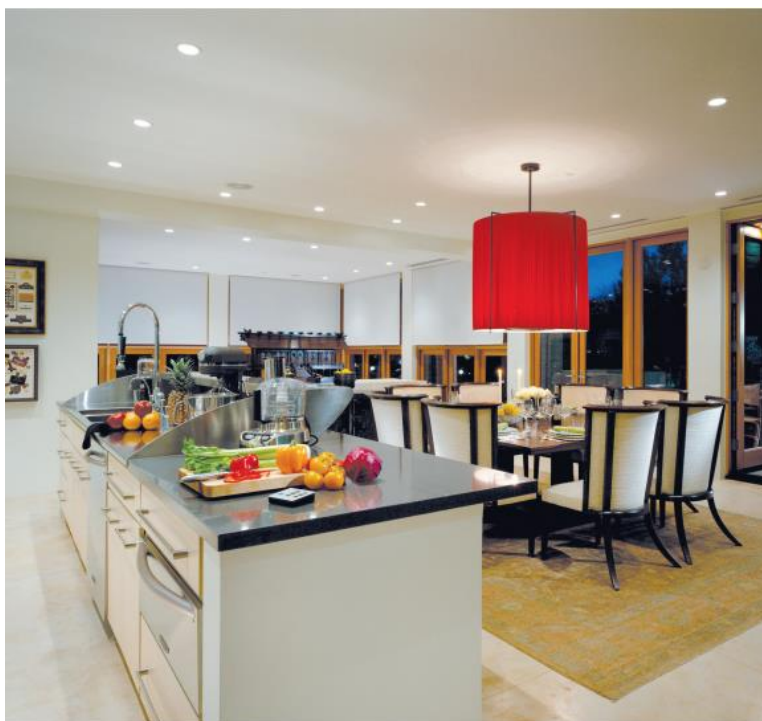
Figure 6-1 Recessed Downlight Luminaires in Ceiling
