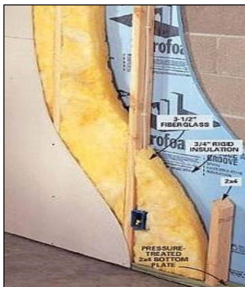
Figure 3-29: Masonry Wall With Furring Details
