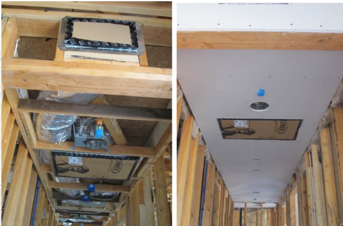
Figure 4-11: Ducts Routed Through a Dropped Ceiling
