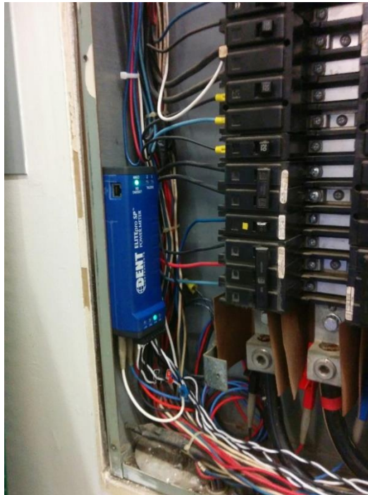
Figure 2: In-Panel Electrical Metering Setup with DENT ElitePro Logger at Mills College
