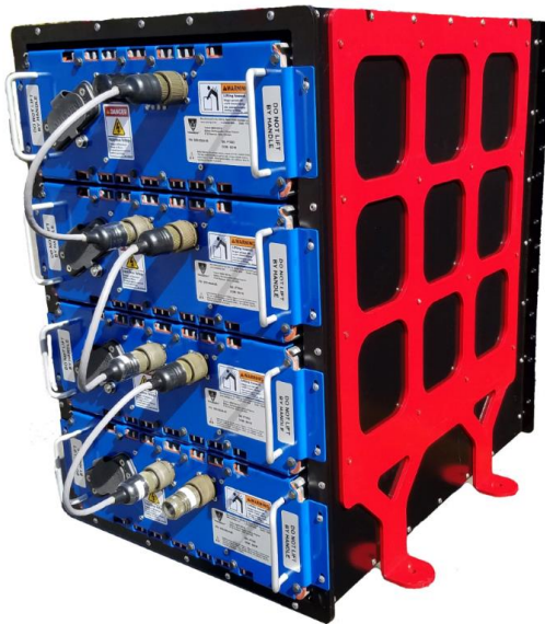
Figure 3: Battery System as Installed
