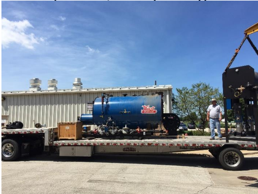
Figure 28: Complete Boiler/Burner System Shipped to Host Site
