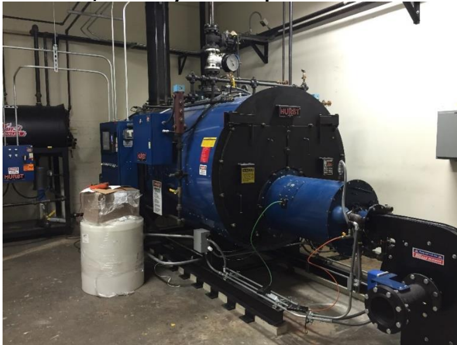
Figure 30: Boiler/Burner System Complete Installation at Host Site
