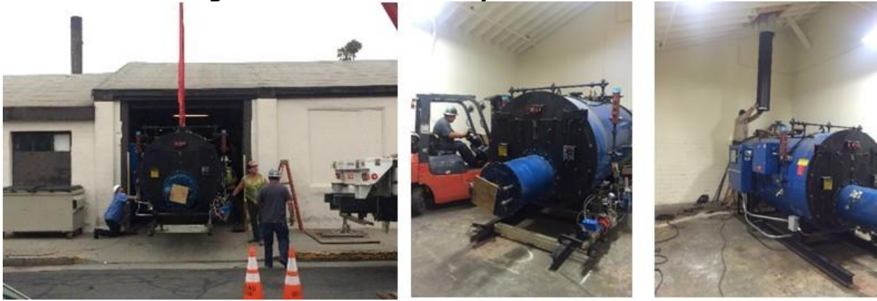
Figure 29: Installation Sequence at Host Site
