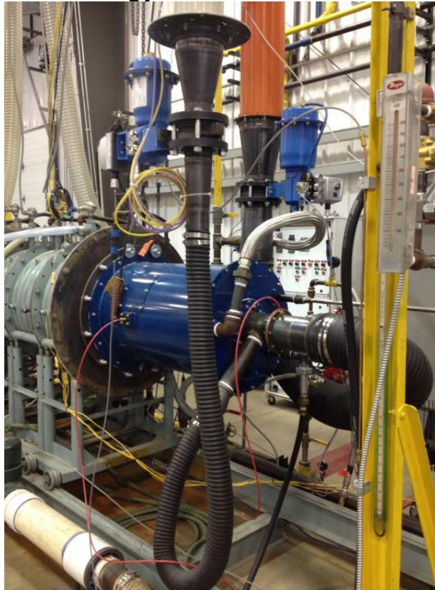
Figure 7: Prototype Dynamic Staged Entrainment Burner Installed on Gas Technology Inc.'s Boiler Simulator Facility
