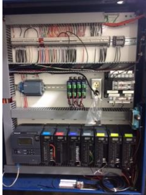
Figure 31: Honeywell Slate Controls with various Modules at the Bottom
