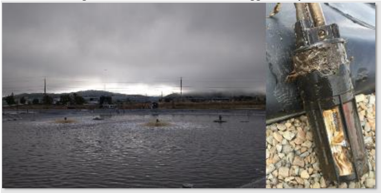
Photograph of source water pond (Left) and clogged feed submersible pump (right)
