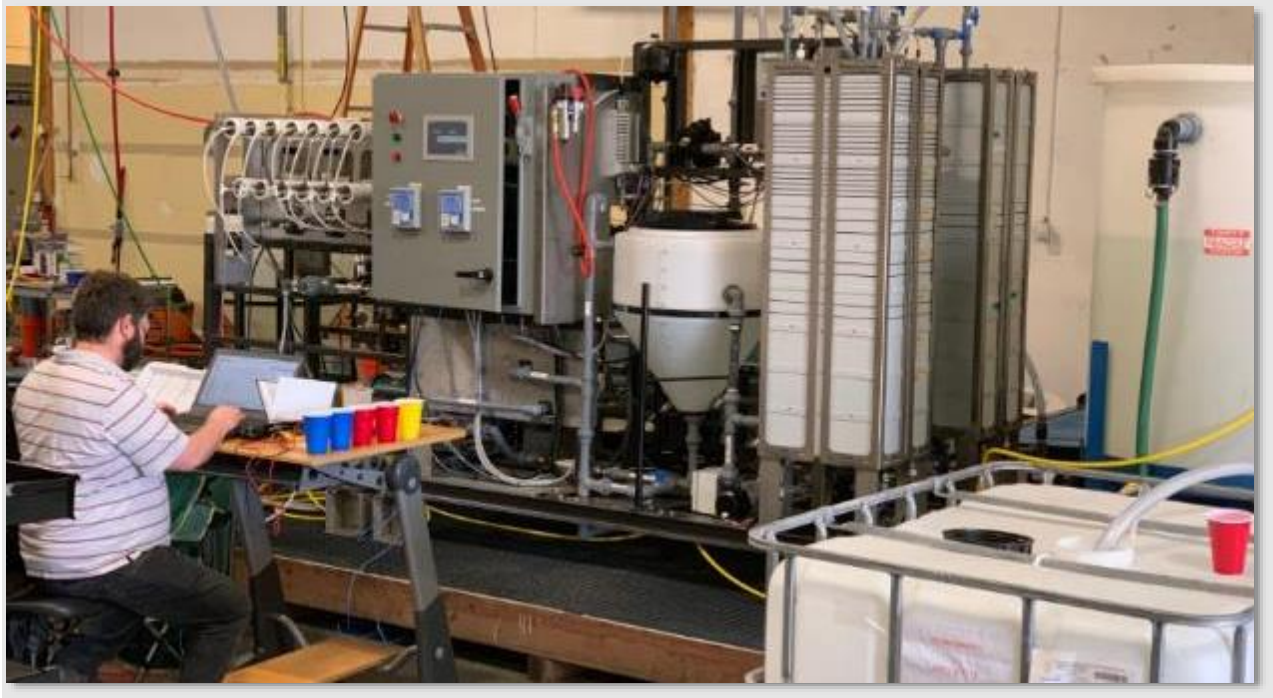
Pictures of the PFO Recycler 2 Skid
