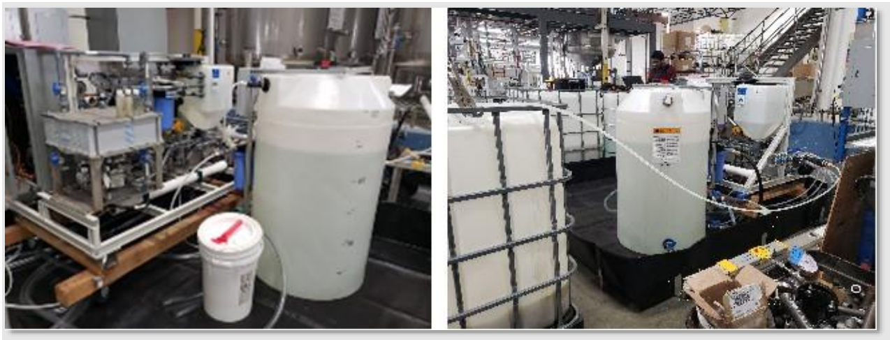
Pictures of the PFO Recycler 1 Skid
