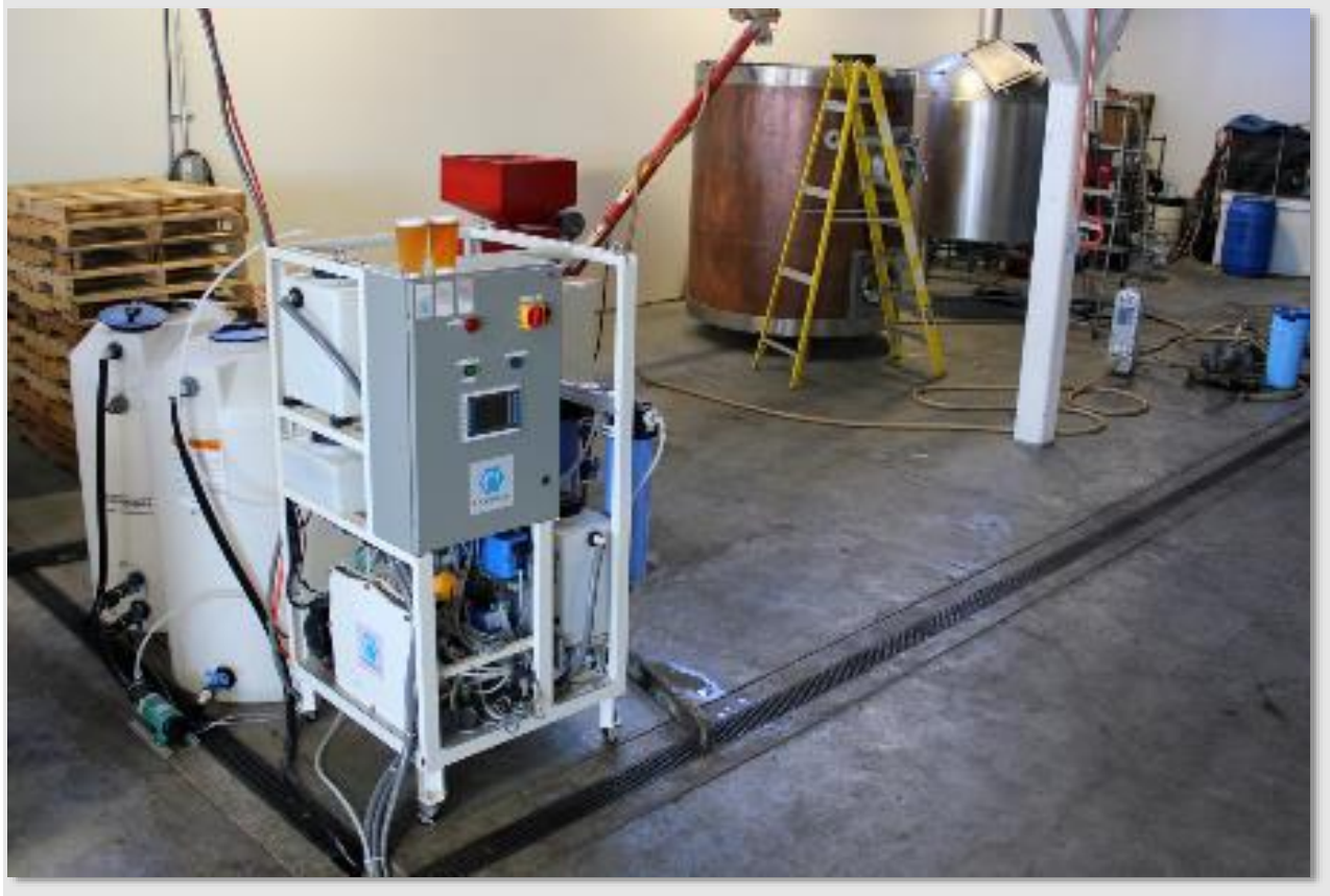
Pictures of the PFO Recycler Skid
