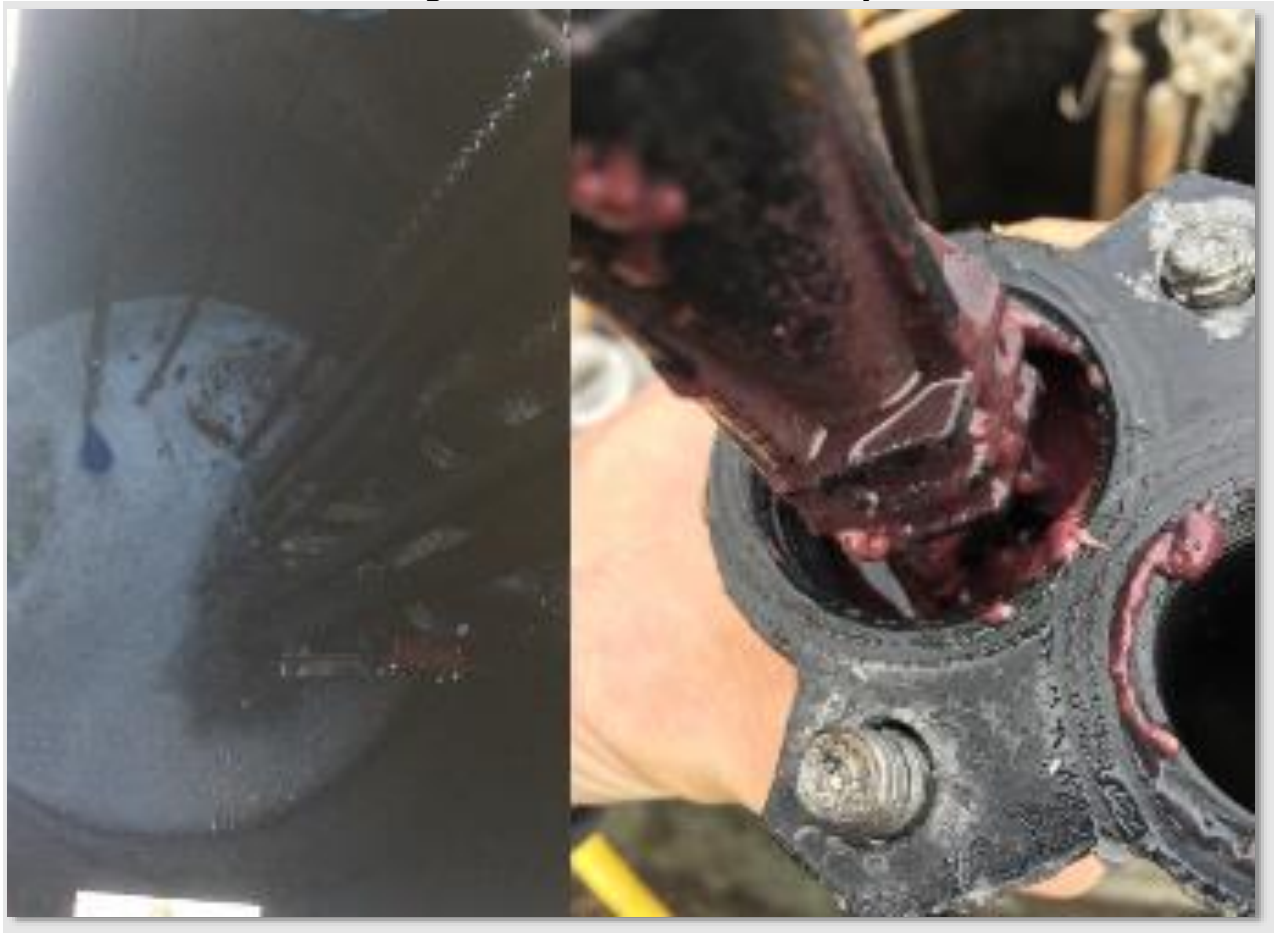
Pictures of source water sump and clogging of sump pump feeding pilot
