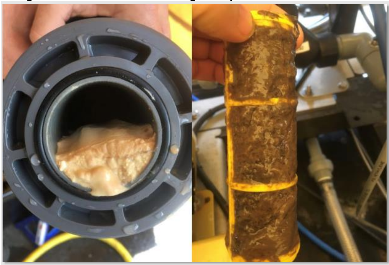
Pictures of biogrowth that clogged feed pipe (left) and pre-strainer (right)
