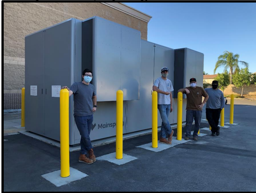
Figure 8: Mainspring Energy's Linear Generator
