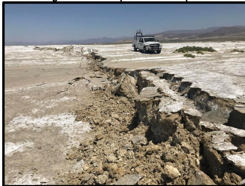
Figure 10: Earthquake Fault Rupture
