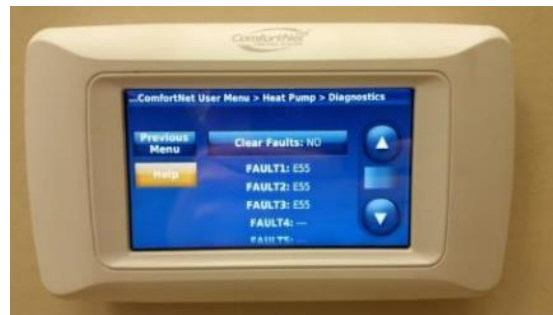
Figure 86: Thermostat Display with High Discharge Temperature Faults
