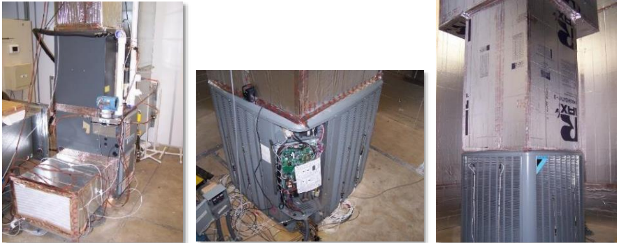
Figure 17: Test Unit Installation
