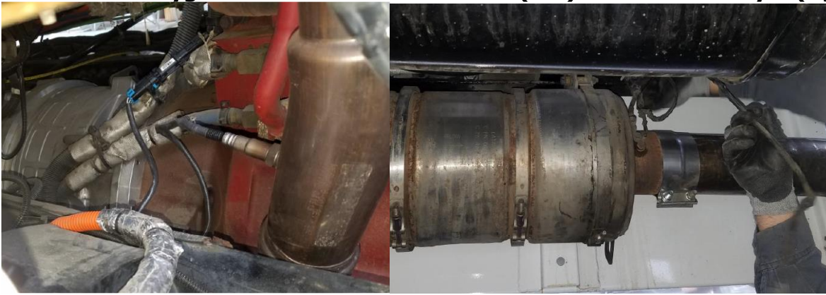
Figure 78: New Oxygen Sensors Installed Before (left) and After Catalyst (right)
