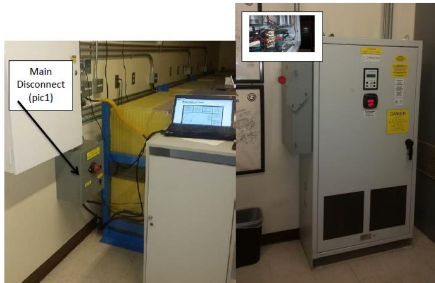
Figure 72: Main Power Cabinets, Batteries and Controls Near the Engine Dyno
