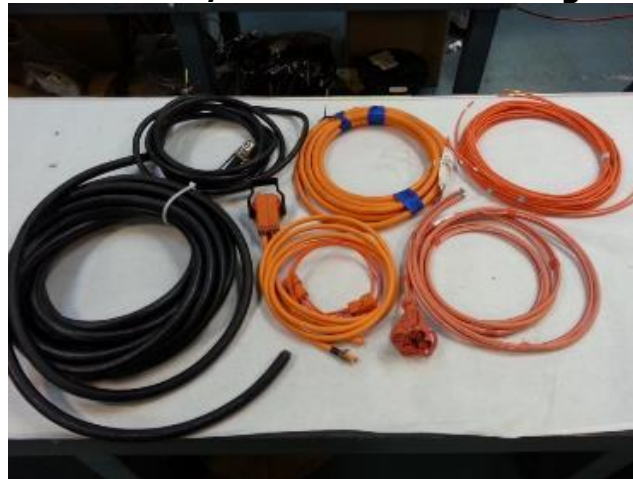
Figure 43: Power/ HV Cables and Wiring Harness
