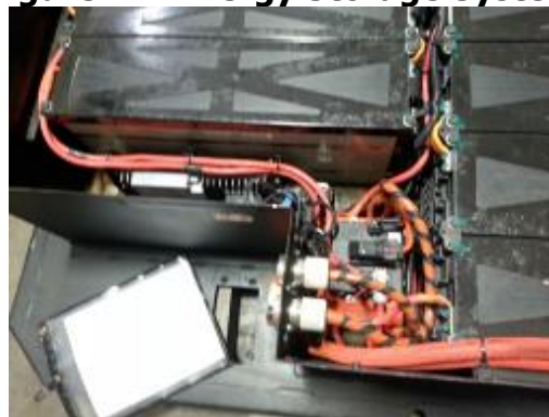
Figure 41: Energy Storage System
