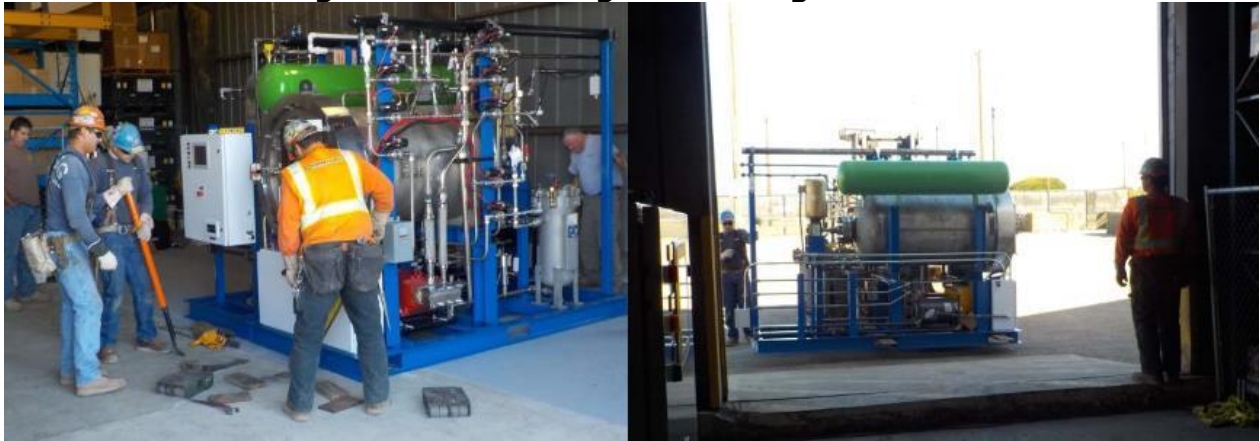
Figure 10: Receiving and Setting Machine
