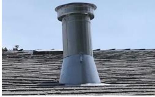
Figure A-7: Roof Vent for Smart Residential Ventilation System
