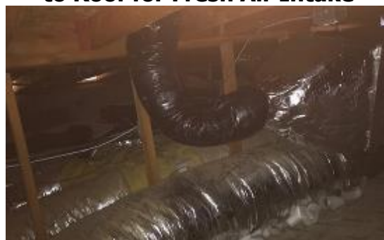
Figure A-6: Smart Residential Ventilation Duct Connections from Fan Box to Roof for Fresh Air Intake
