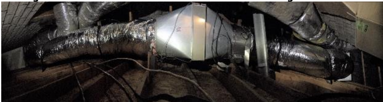
Figure A-10: Filter Box Installed in Outside Air Ducting in East Home
