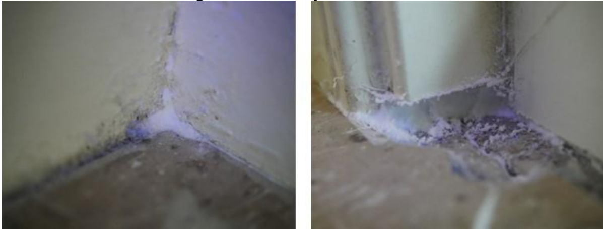
Seals formed at baseboards (left) and at bottom of sliding door frame (right)
