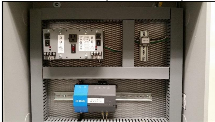
Figure 6: Tridium Building Automation System JACE
