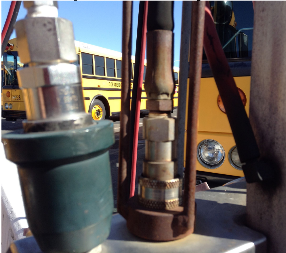
Figure 6: Rust around Fueling Post
