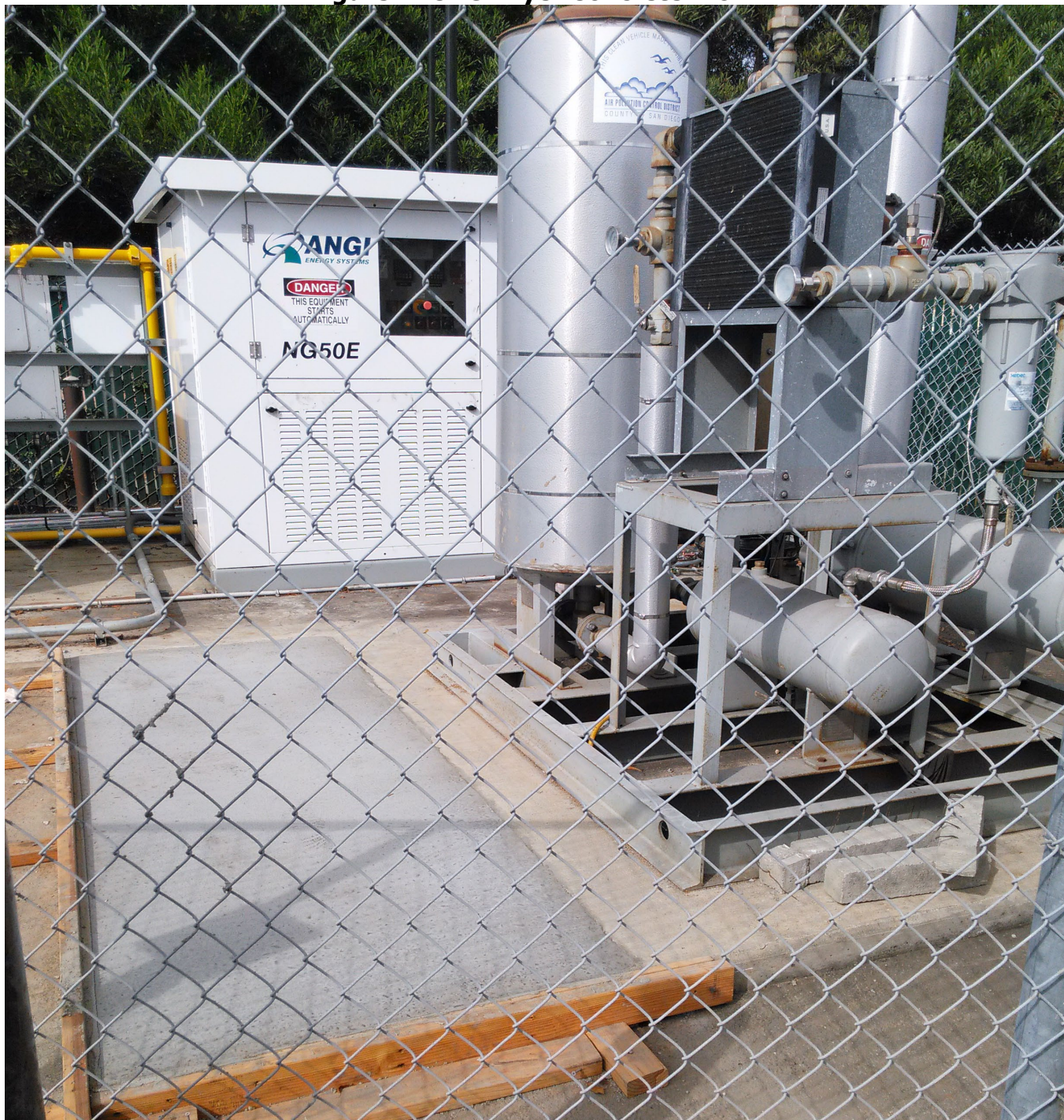
Figure 1: CNG Dryer Concrete Work
