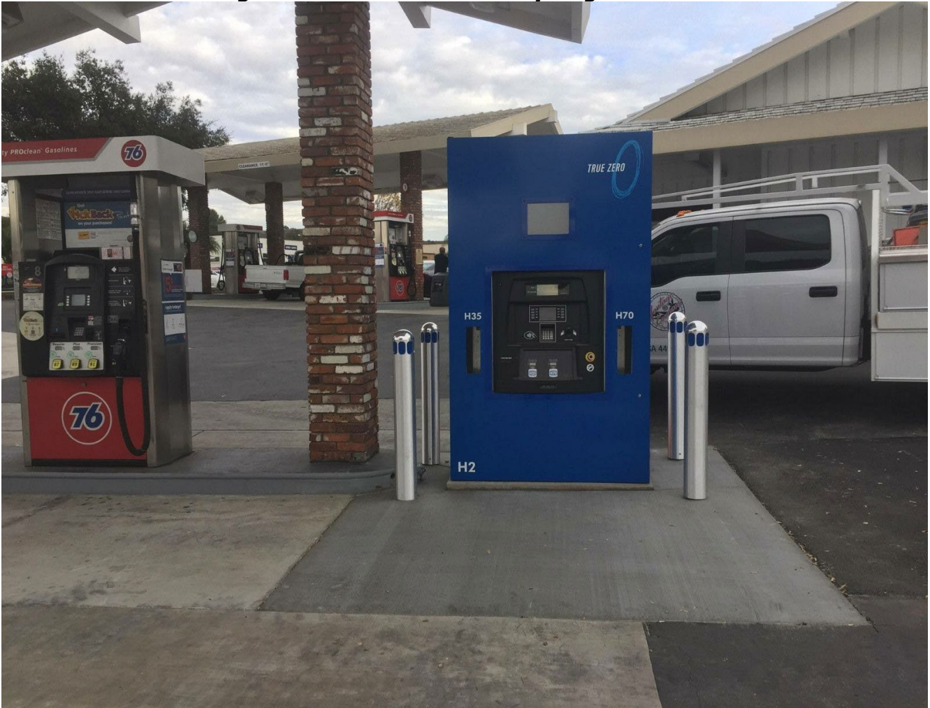
Figure 10: Thousand Oaks Hydrogen Station
