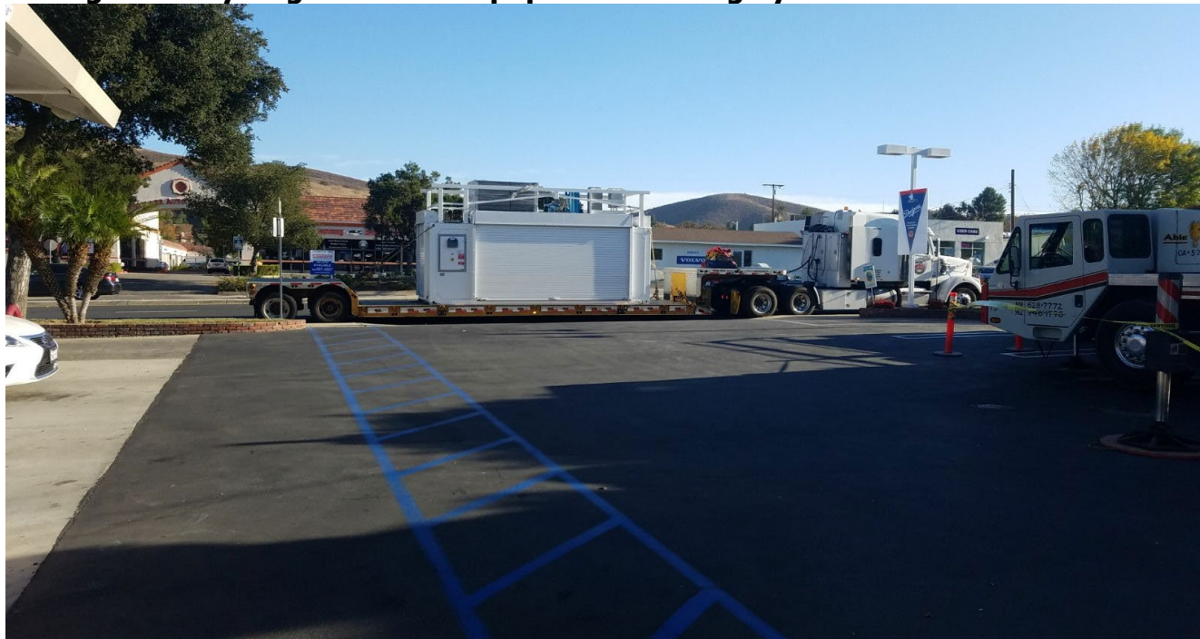
Figure 5: Hydrogen Station Equipment Arriving by Truck in Thousand Oaks.
