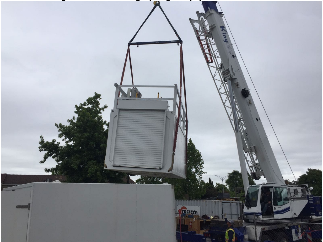
Figure 5: Crane Lifting Hydrogen Equipment in Fremont
