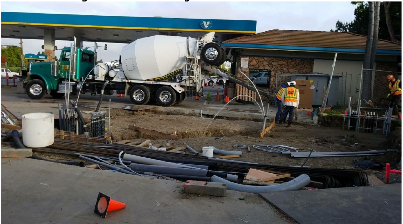
Figure 4: Photo Showing Station Under Construction.
