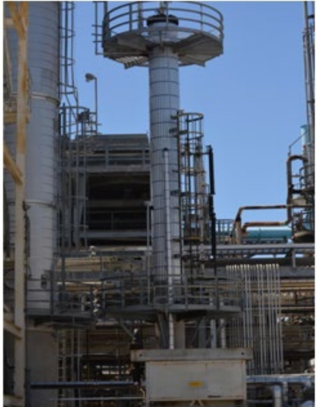
Figure 13: Reworked Support Units Including Caustic Scrubber, Sidecut Stripper, Caustic burner, and SOX Burner Unit.
