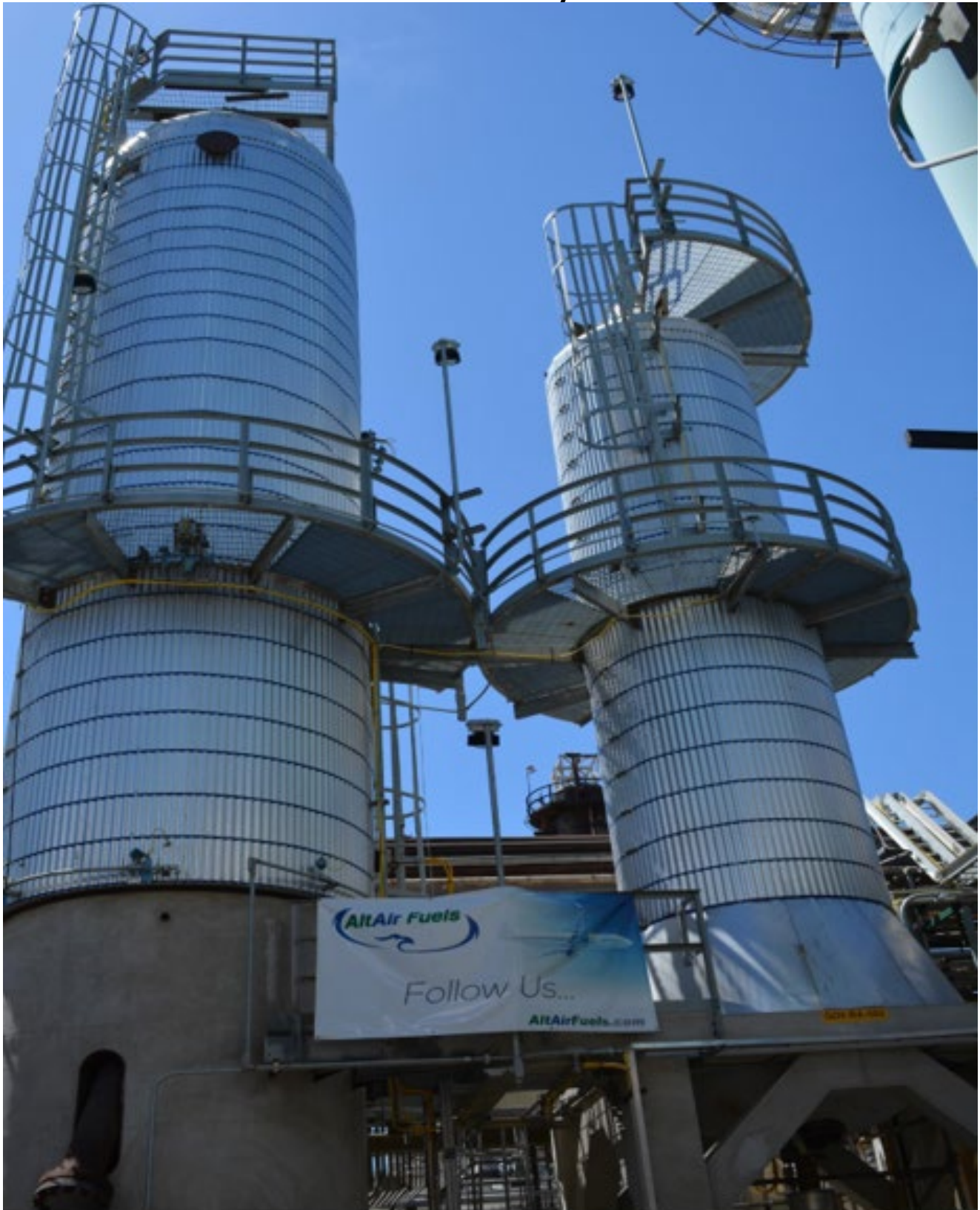
Figure 5: Installed New Reactors with New Internals and Temperature Thermometry
