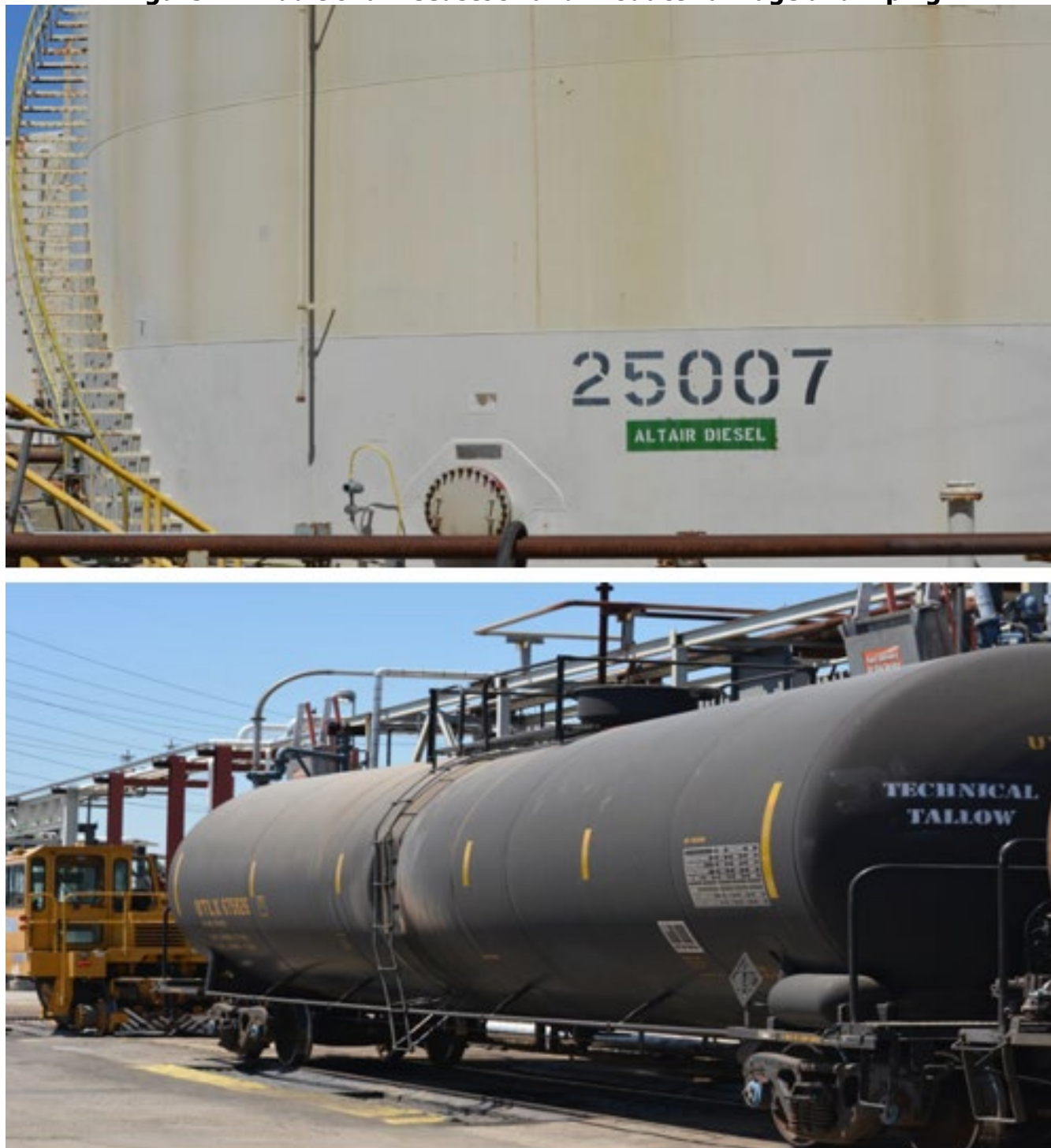
Figure 14: Additional Feedstock and Product Tankage and Piping
