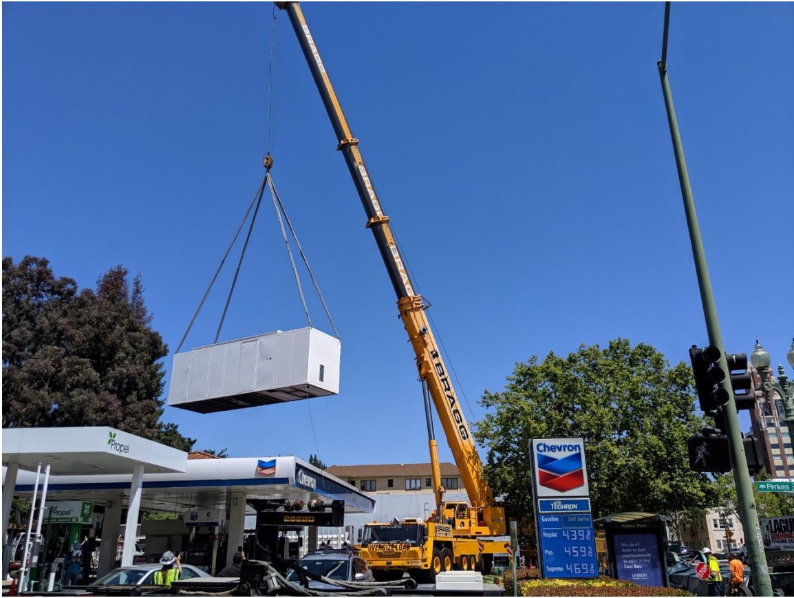
Crane lifting hydrogen compressing and dispensing unit off delivery truck in Oakland
