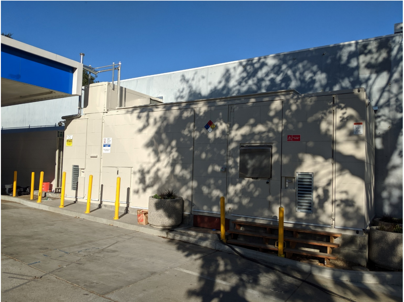
Figure 4: Installed Linde Unit (Compressing and Dispensing Equipment)
