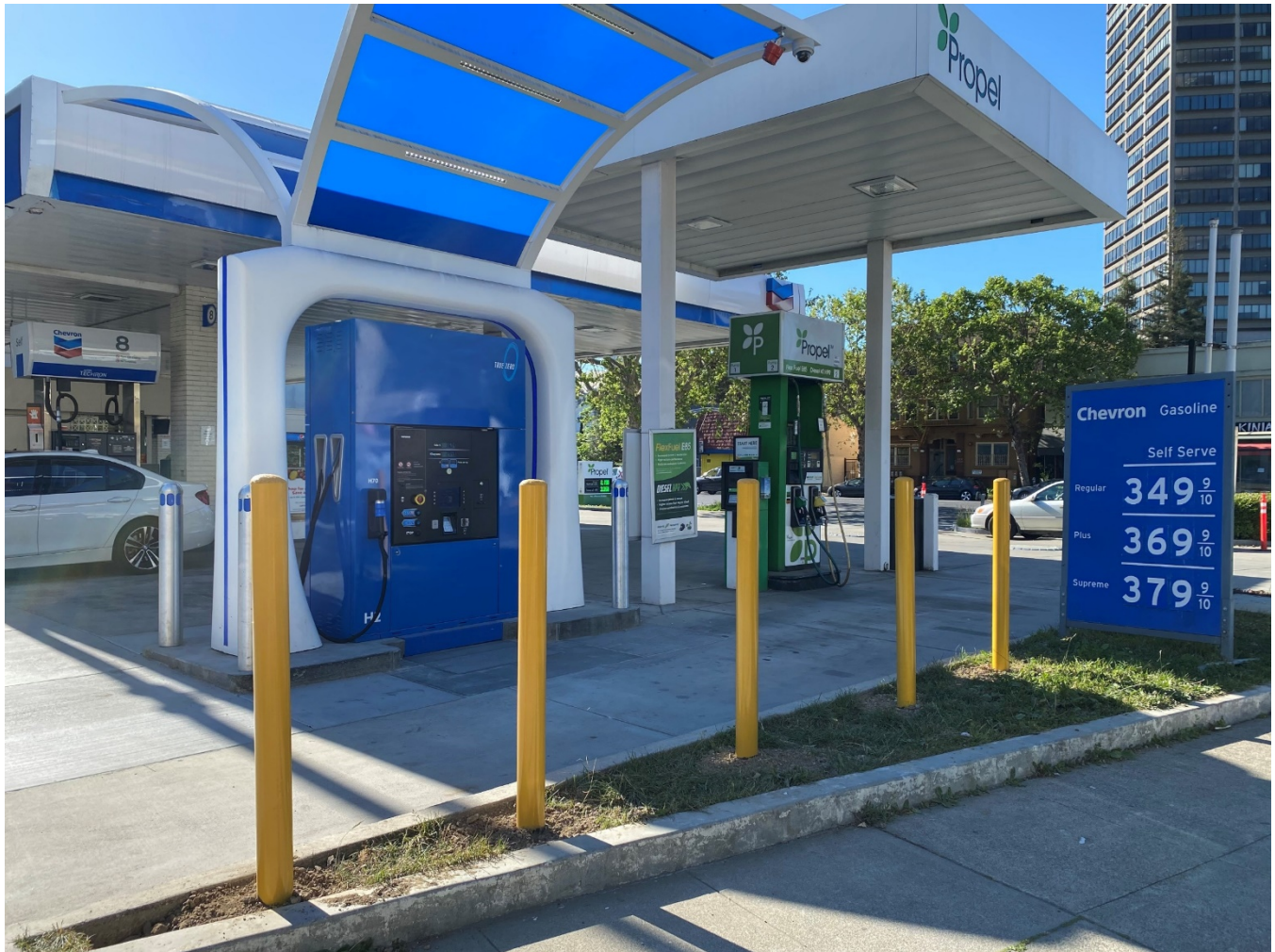
Figure 3: Installed Tatsuno Dispenser with two Fueling Positions
