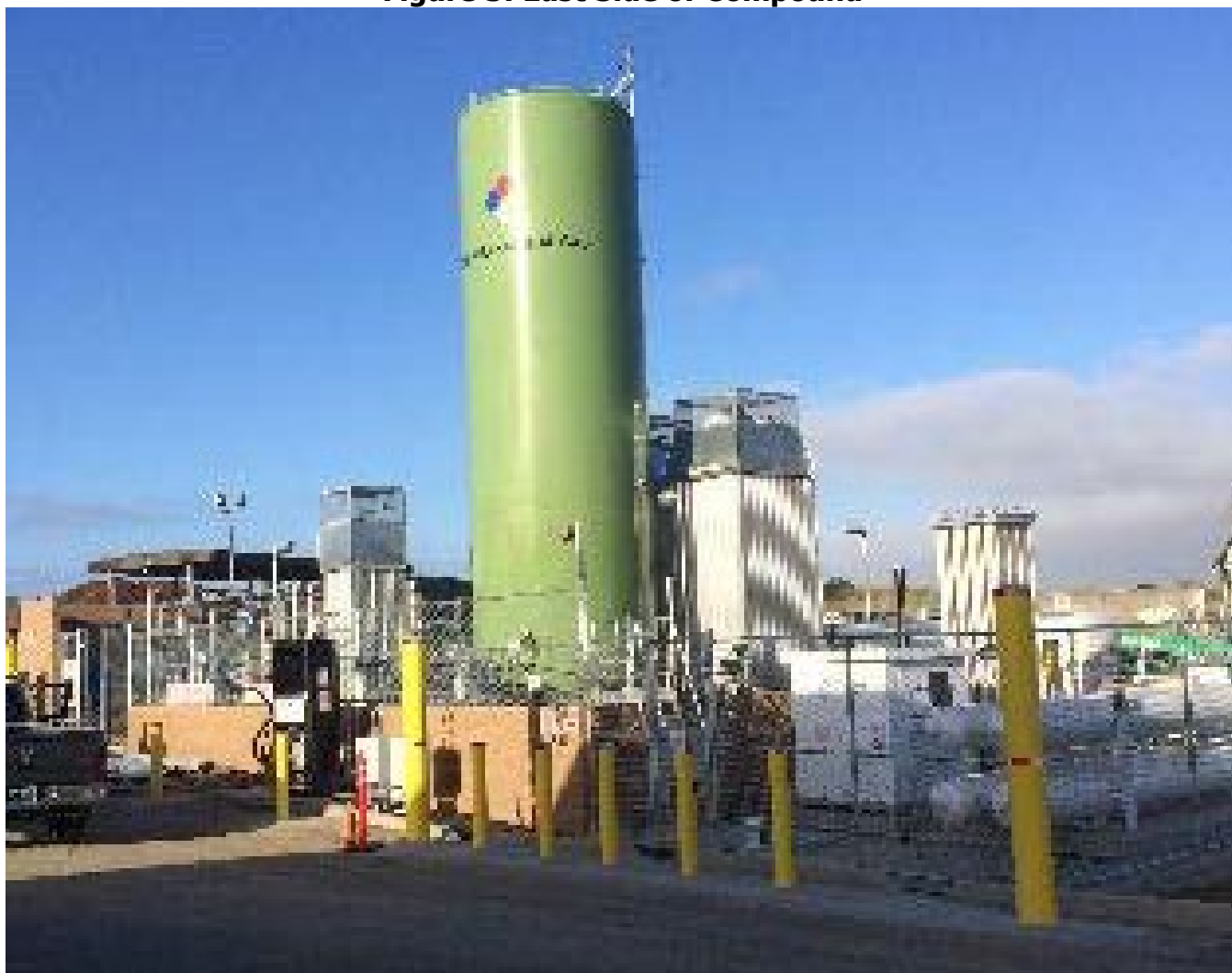
Figure 3: East Side of Compound
