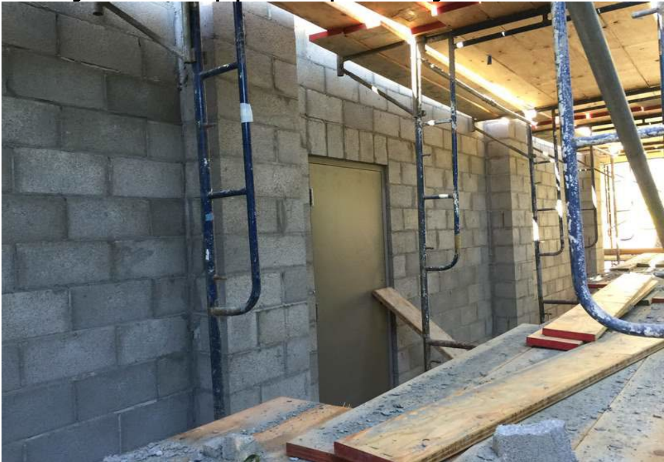
Figure 5: Station Equipment Compound During Cement Block Work
