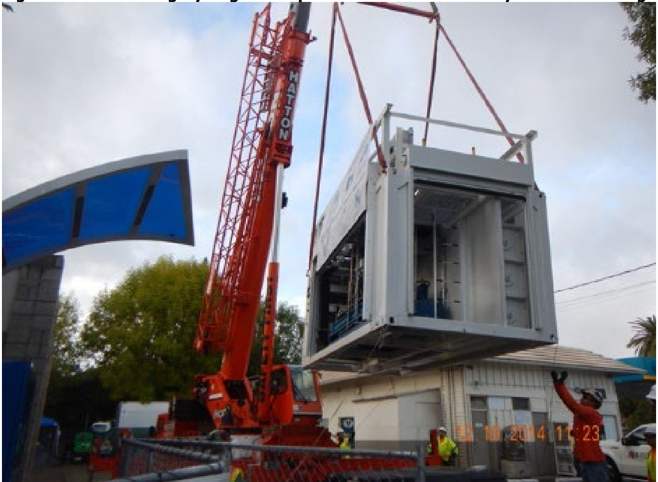
Figure 6: Crane Lifting Hydrogen Compressor Skid Off of Delivery Truck in Saratoga
