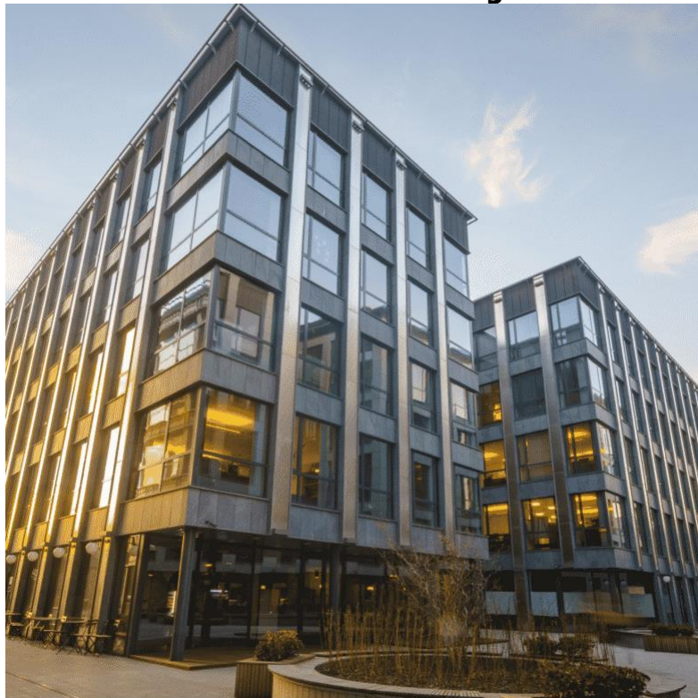
Figure 2: Ubiquitous Energy's Transparent PV Window Coating Installed on a Commercial Building
