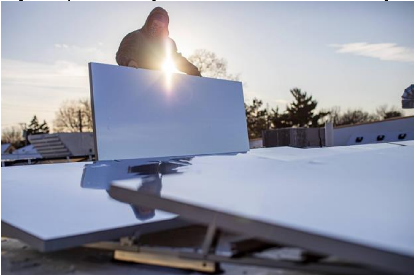
Figure 3: SkyCool Panels Being Mounted with Conventional Solar Panel Racking
