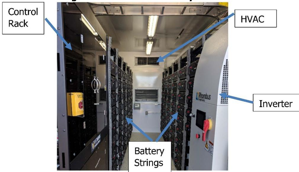
Inside the ESS container. Left: Control and high voltage switching rack. Right: Inverter. Back: Battery racks
