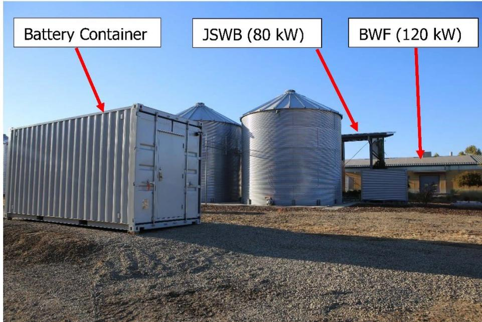
Photo of the microgrid showing the battery system in a 20ft shipping container, the Jackson Sustainable Winery Building, and the Brewery Winery and Food Science Building.
