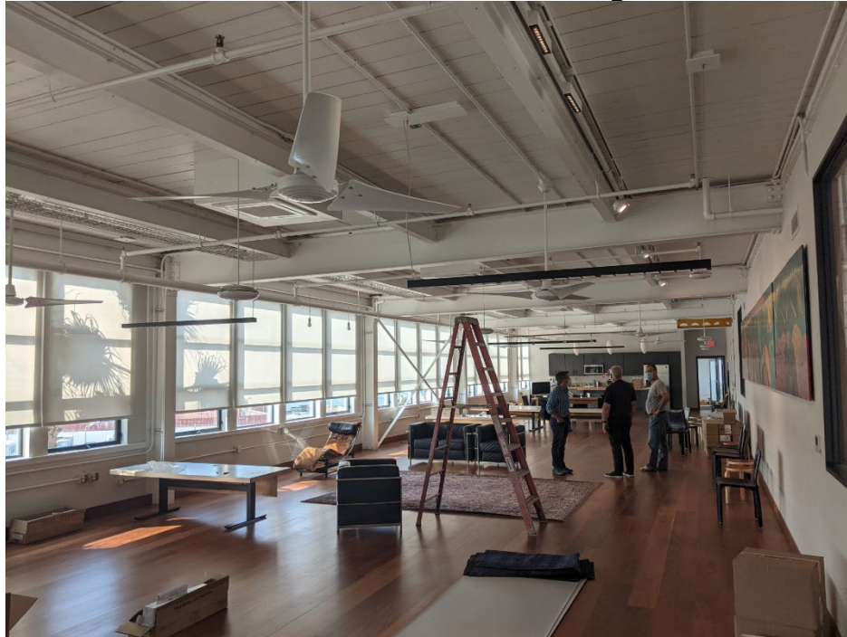
Figure 10: Office of Loisos + Ubbelohde During Fixture Installation
