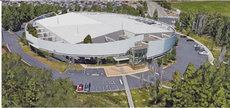
Figure 7: Kaiser Permanente Pleasanton Data Center
