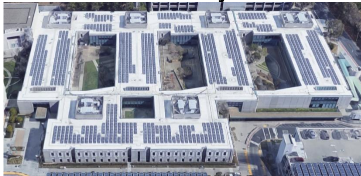
Figure 1: Kaiser Permanente Vallejo Medical Office Building
