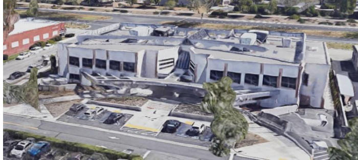
Figure 2: Kaiser Permanente Whittier Medical Office Building
