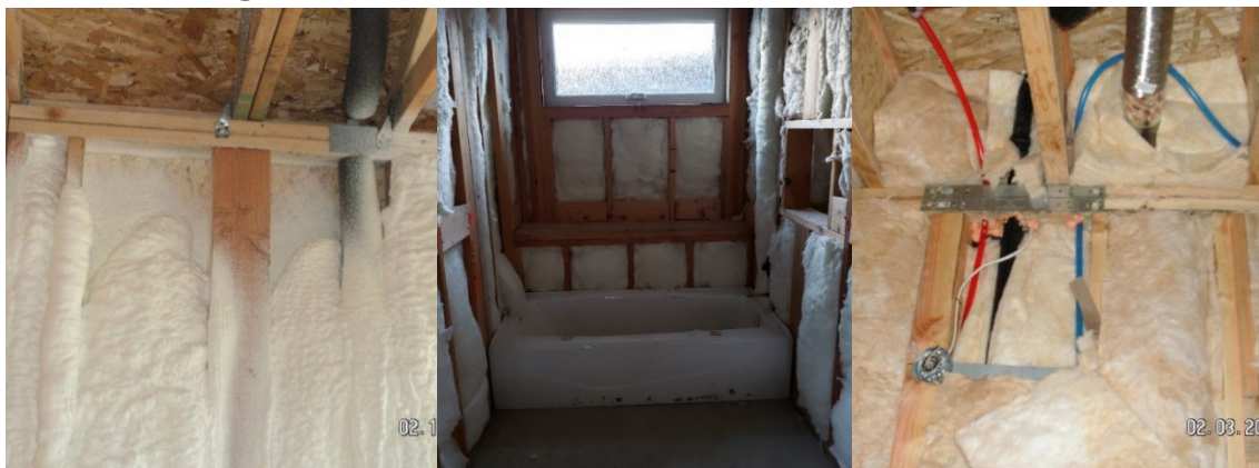
Figure 22: Deficiencies in Insulation Installation
