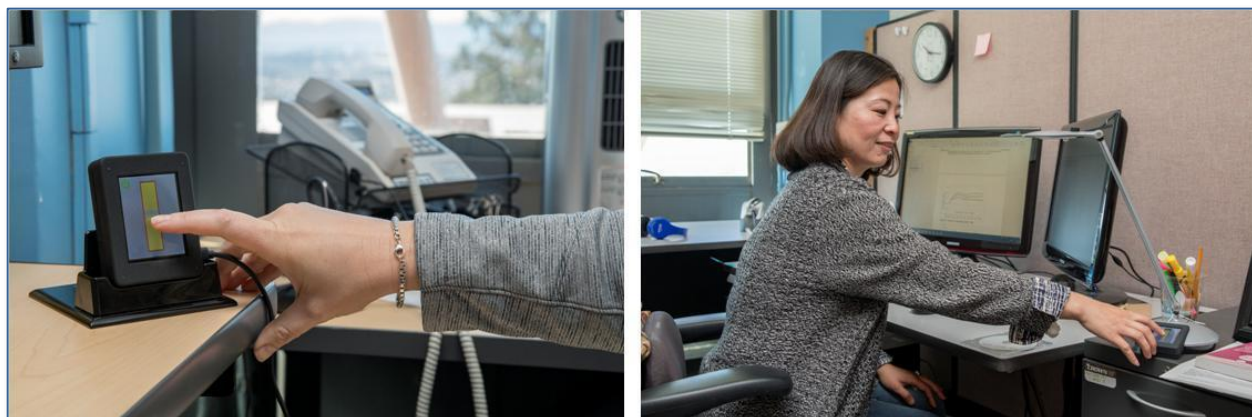
Figure 19: Field Test #2 Included Desktop (left), and Task Lamp-Integrated (right) Readings-At-Desk Controller Versions
