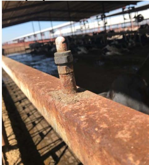
Figure 4: Pen Sprayer Header with Example Nozzle
