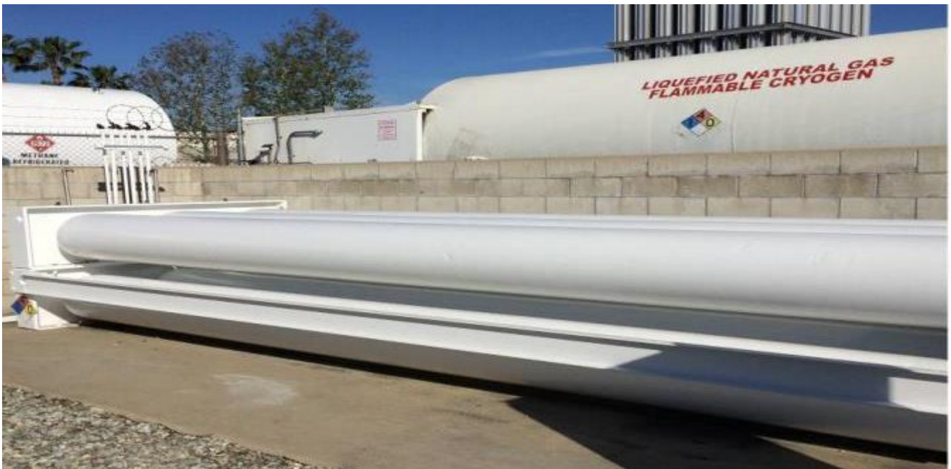
Figure 6: CNG Vessels Corrosion Control and Paint
