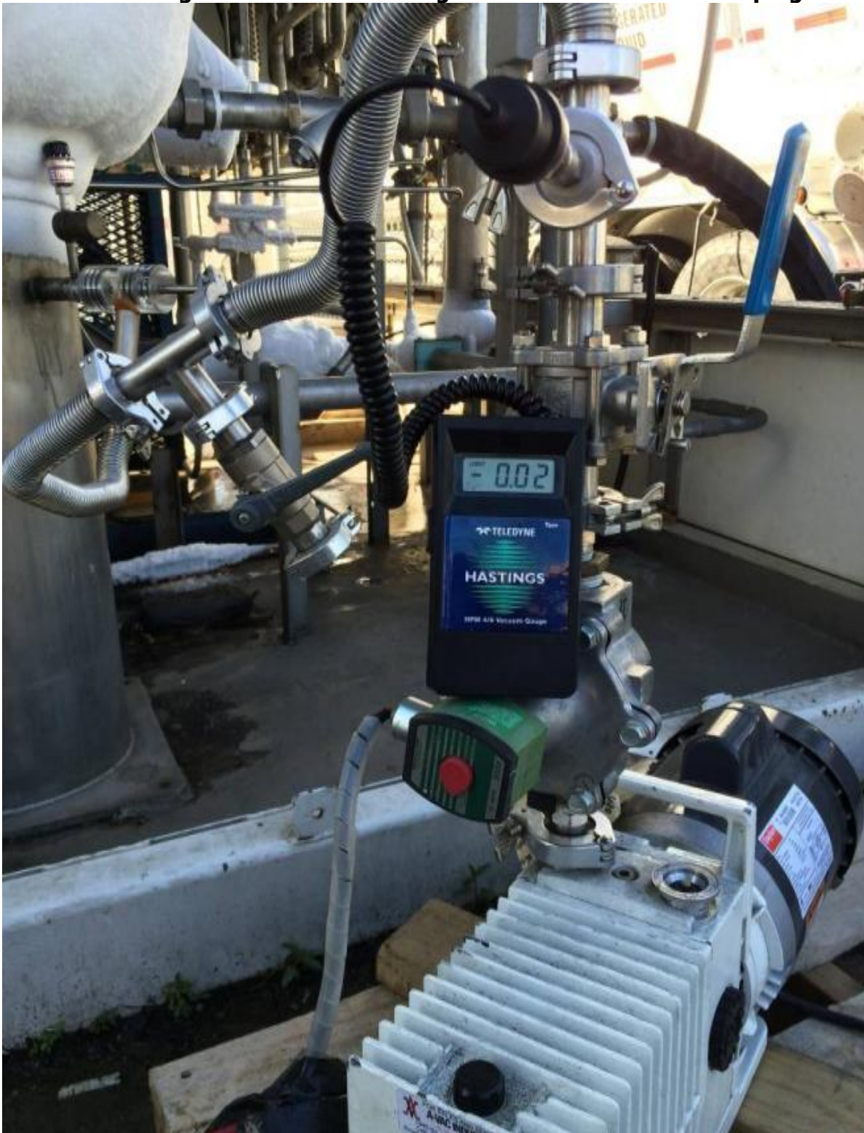
Figure 9: Vacuum Testing LNG Tank and Jacketed Piping
