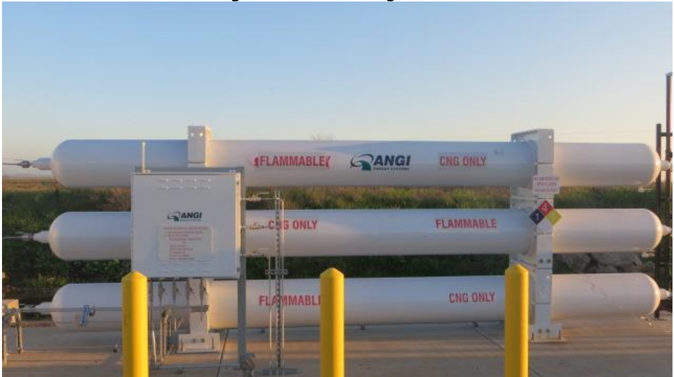
Figure 12: CNG Storage Tanks
