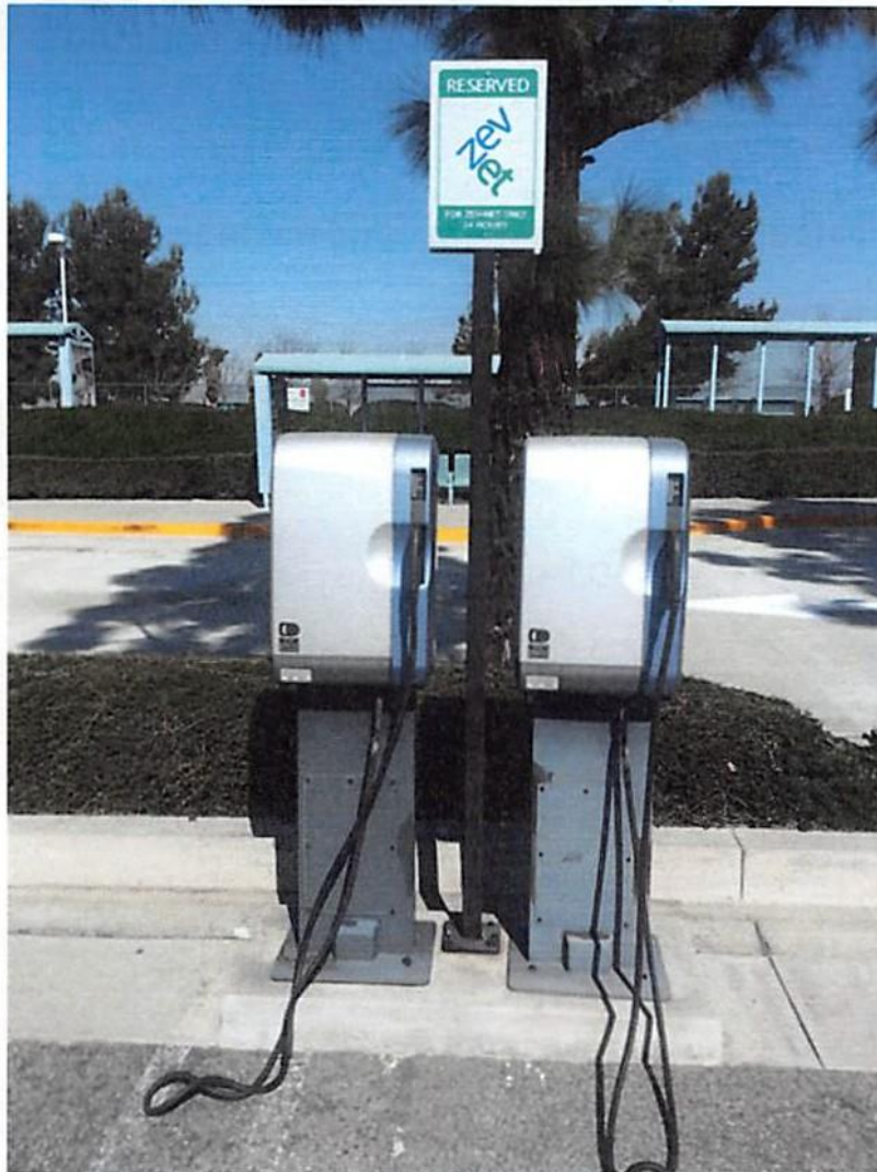
Figure 4: Irvine Train Station Single Port Inductive Charging Stations
