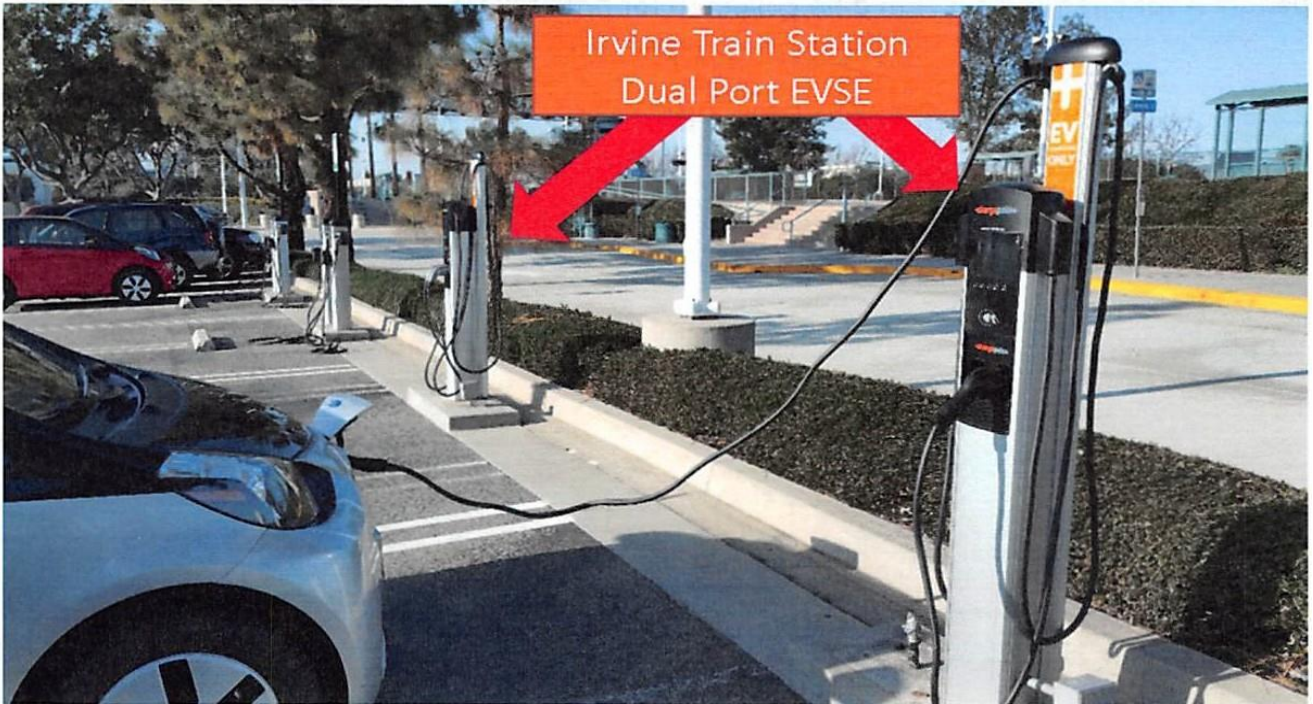
Figure 5: Irvine Train Station Site Post-Installation of Dual-Port Level 2 Chargers
