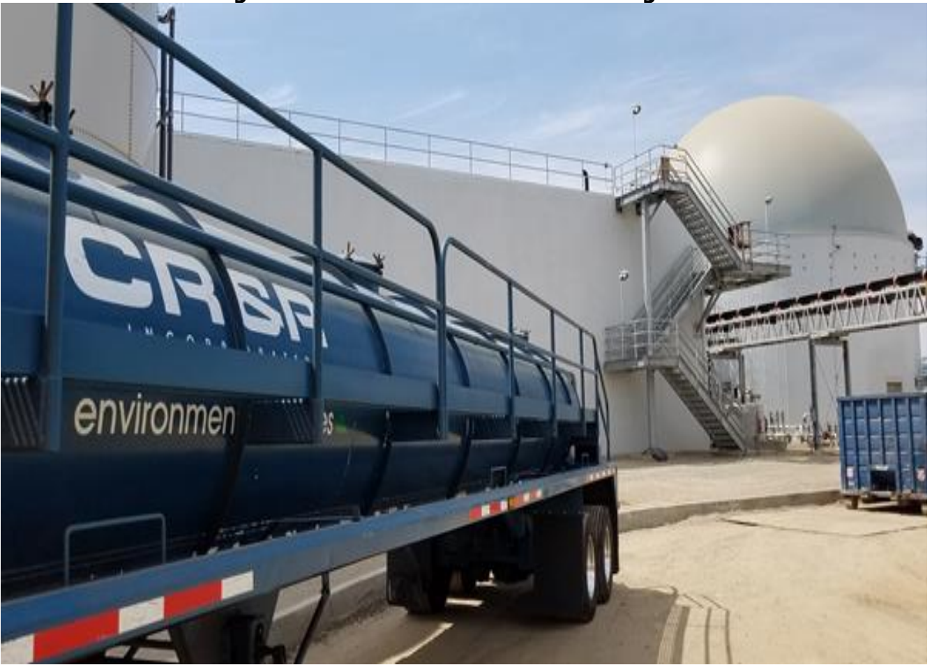
Figure 9: CR&R's Phase I Anaerobic Digester
