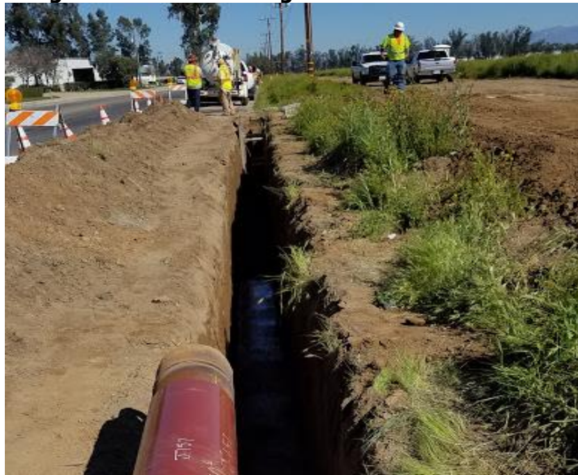
Figure 4: Gas line Being Installed in the Ground
