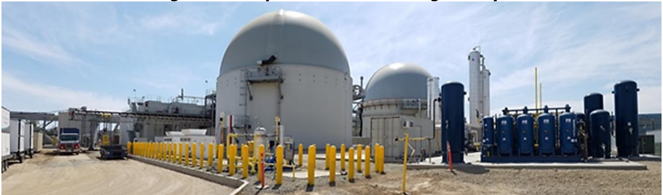
Figure 3: Completed Phase I Fueling Facility
