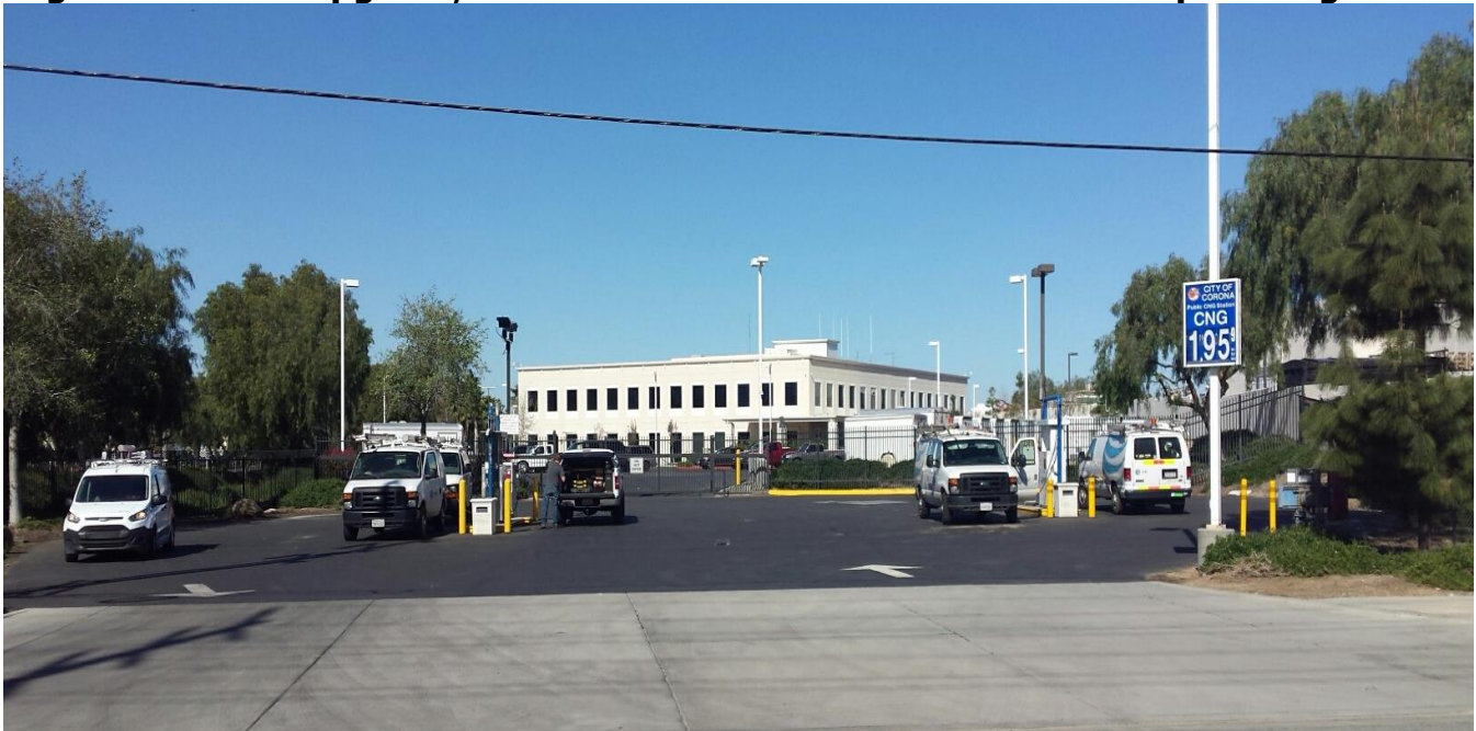
Figure 5: Before upgrade, there would have been 3-4 vehicles deep waiting to fuel
