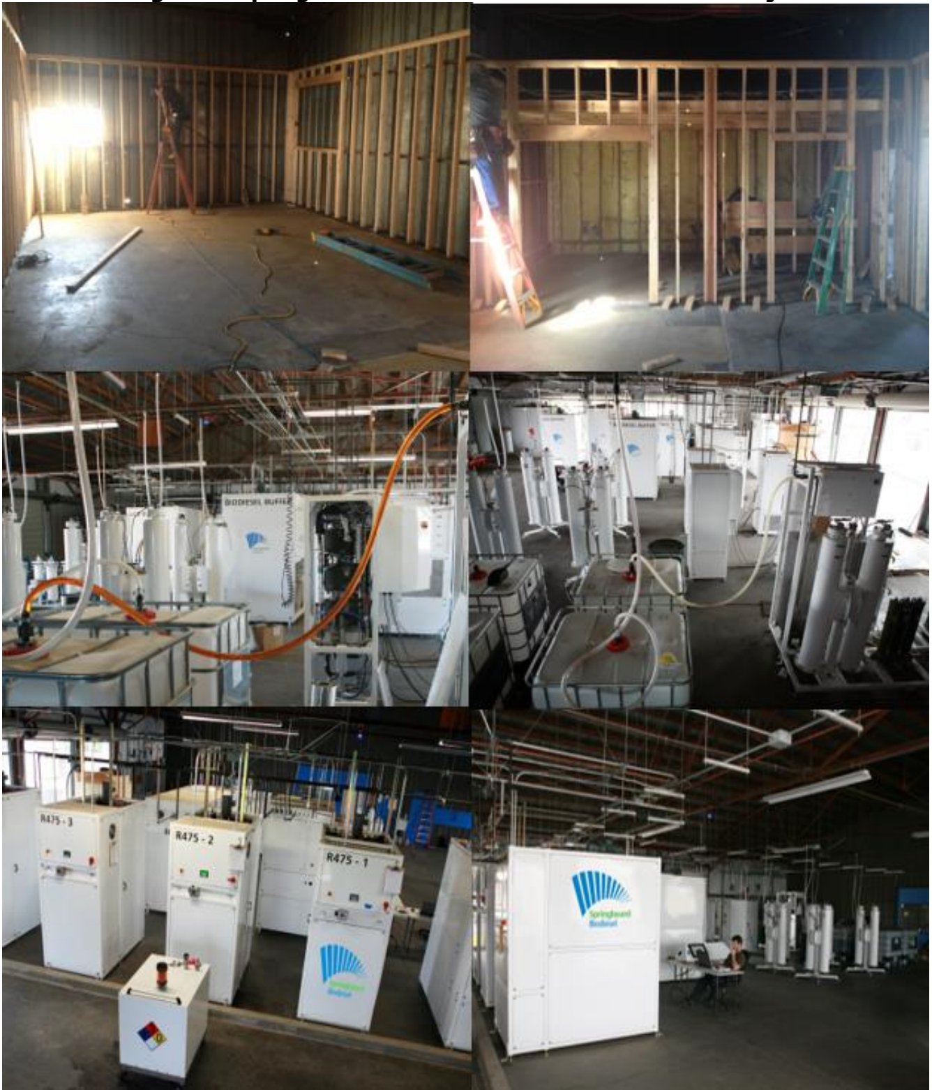
Figure 2: Springboard Biodiesel After the Start of the Project
