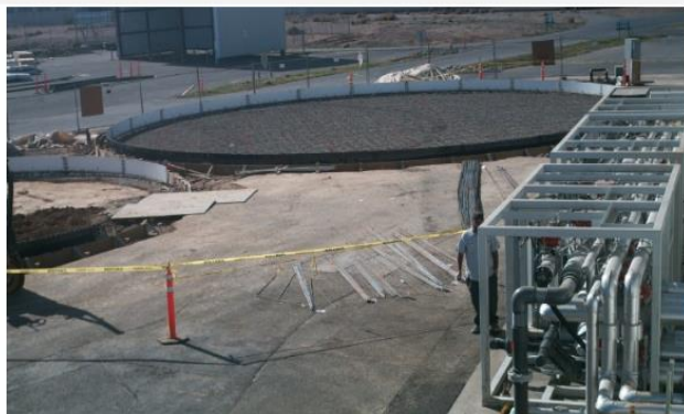
Installing tank starter ring (1.30.14)
