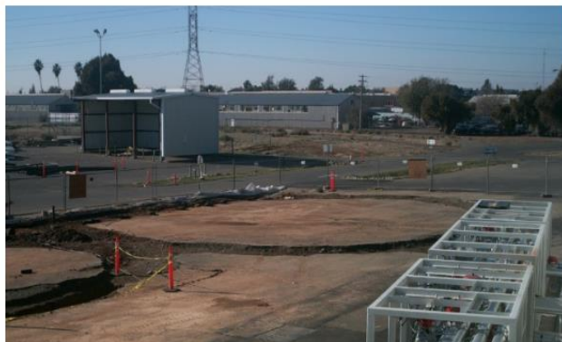
Tank foundation trenching (1.9.14)
