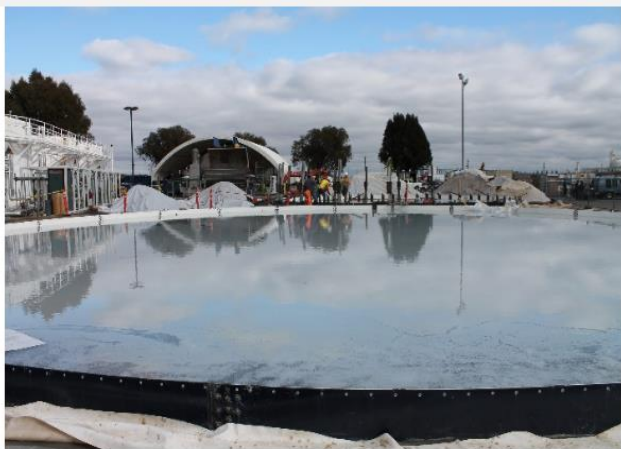
Curing the larger tank floor (2.10.14)
