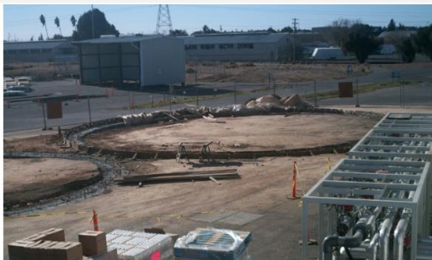
Pouring concrete tank footings (1.21.14)
