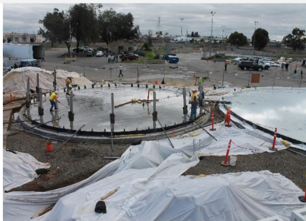
Installing tank wall support scaffold (2.10.14)
