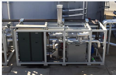
Completed boiler/hot water skid (4.17.15)
