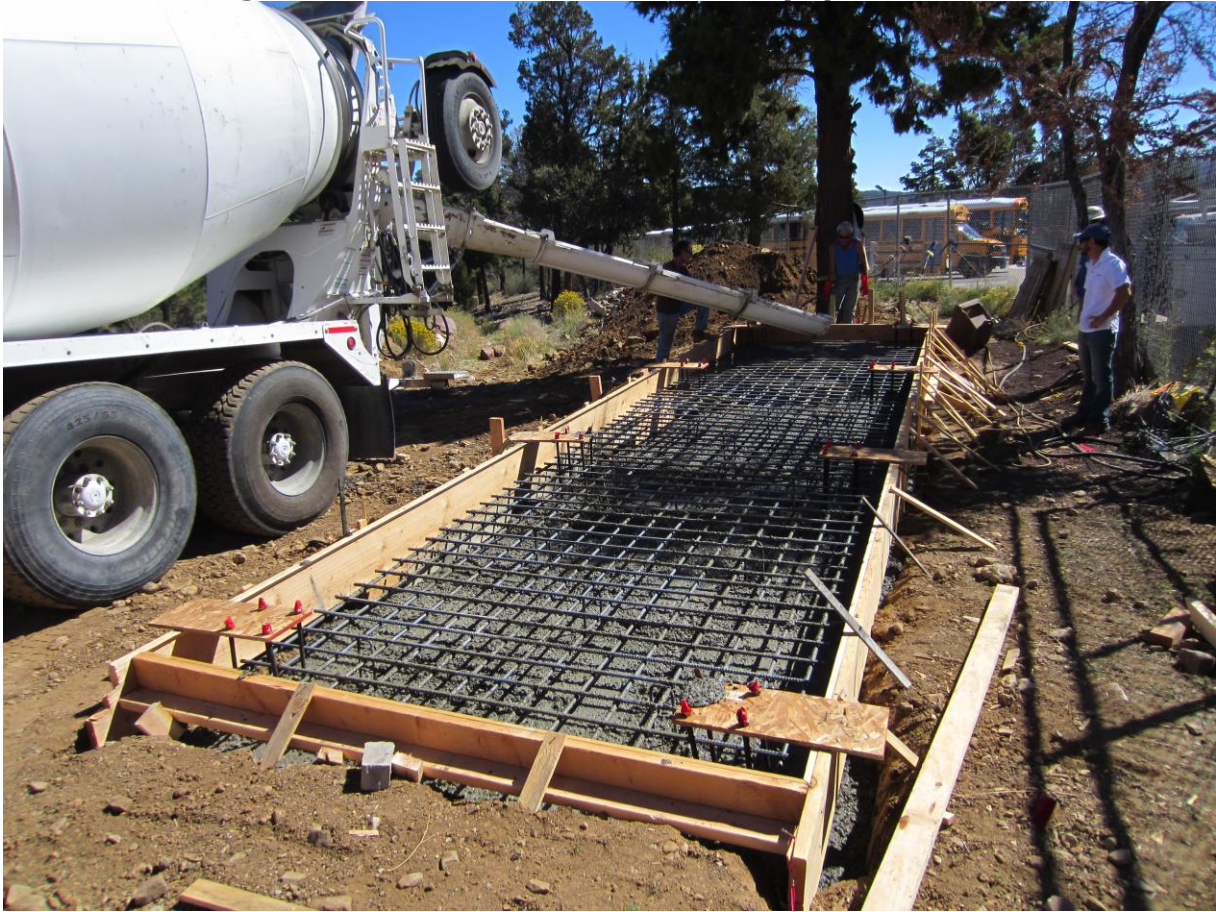
Figure 1: Installation of Concrete Equipment Pad
