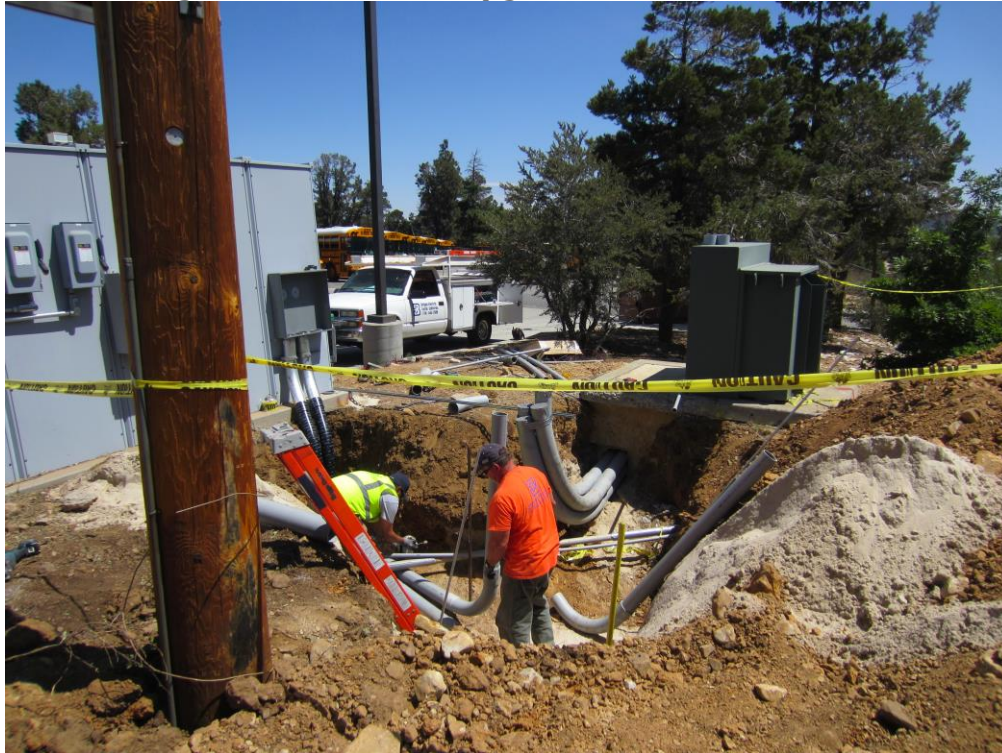
Figure 2: Electrical Upgrades for CNG Station
