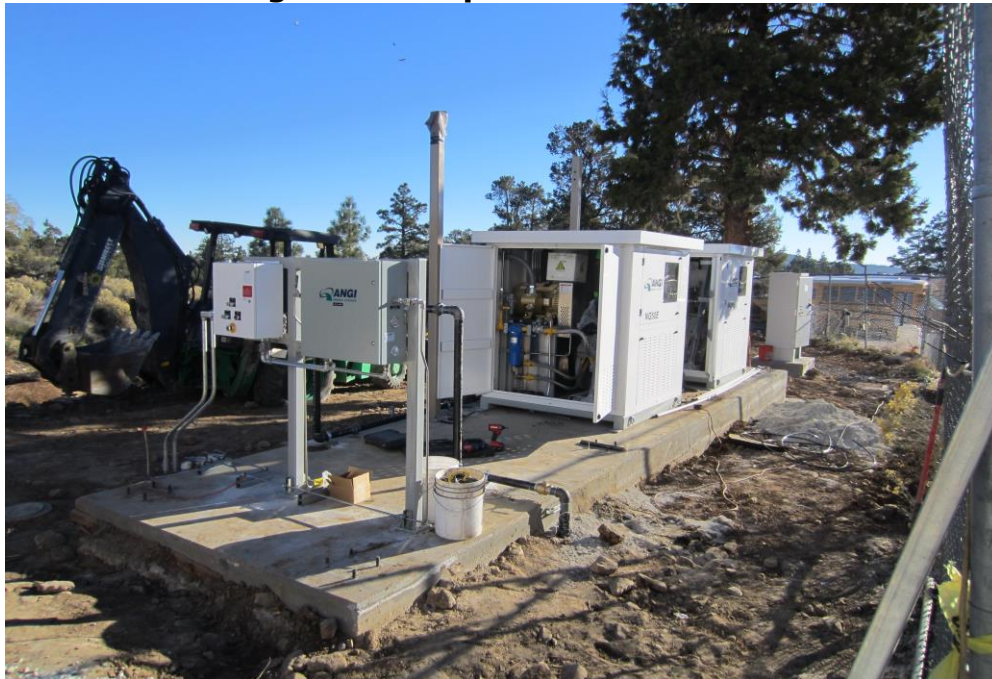
Figure 3: Compressor Installation
